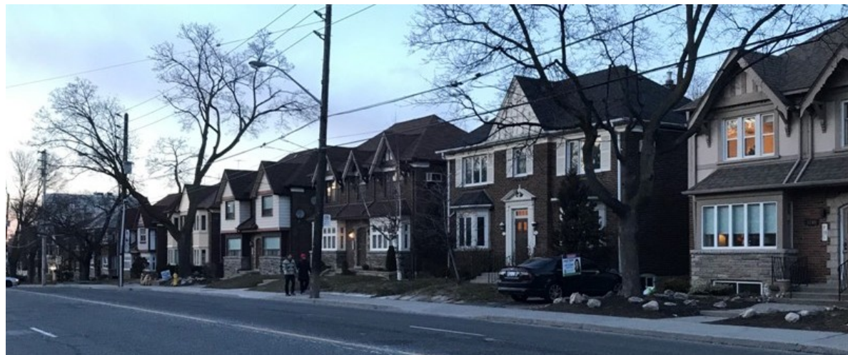
22. 1747-1765 Bayview Avenue, showing the consistency of form and variety of detail in the ten apartment buildings from 1747-1783 Bayview Avenue (HPS, 2018)
