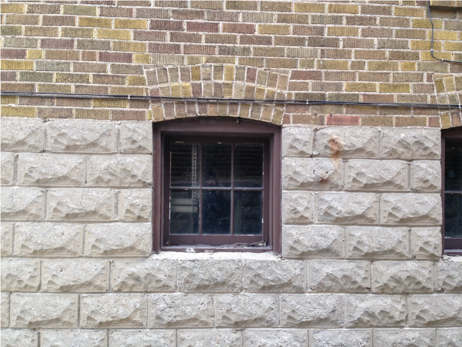
11. Side wall at 1781 Bayview Avenue showing the rusticated concrete block also used at 1783-1785 and the other eight apartment blocks in the sequence. (HPS, 2017)
