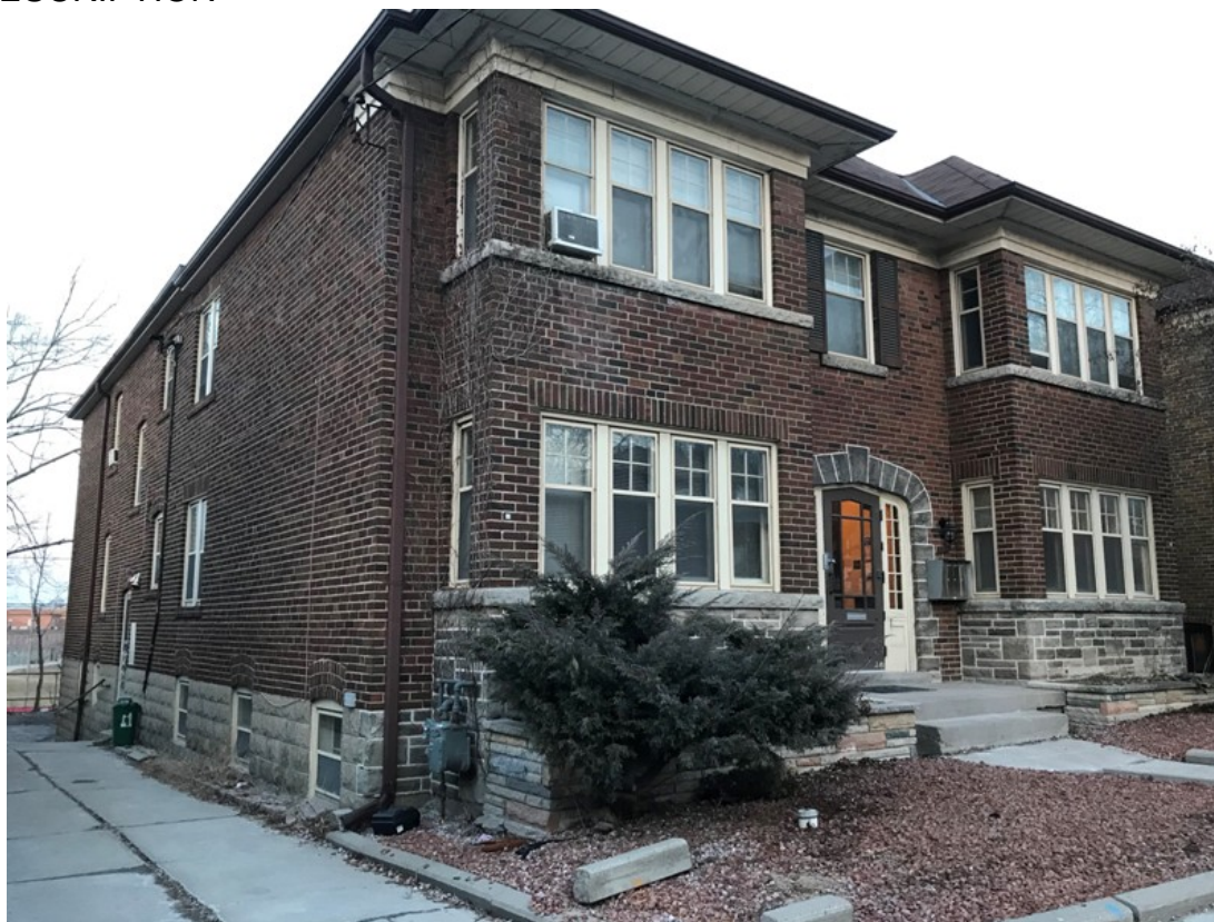
Above: Photograph showing the principal (west) elevation and side (north) elevation of 1783-1785 Bayview Avenue (Heritage Preservation Services [HPS], 2018) Cover: 1783-1785 Bayview Avenue, principal (west) elevation (HPS 2018)
