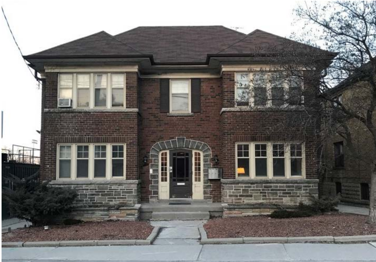
Photograph of the principal (west) elevation at 1783-1785 Bayview Avenue (Heritage Preservation Services (HPS), 2018)
