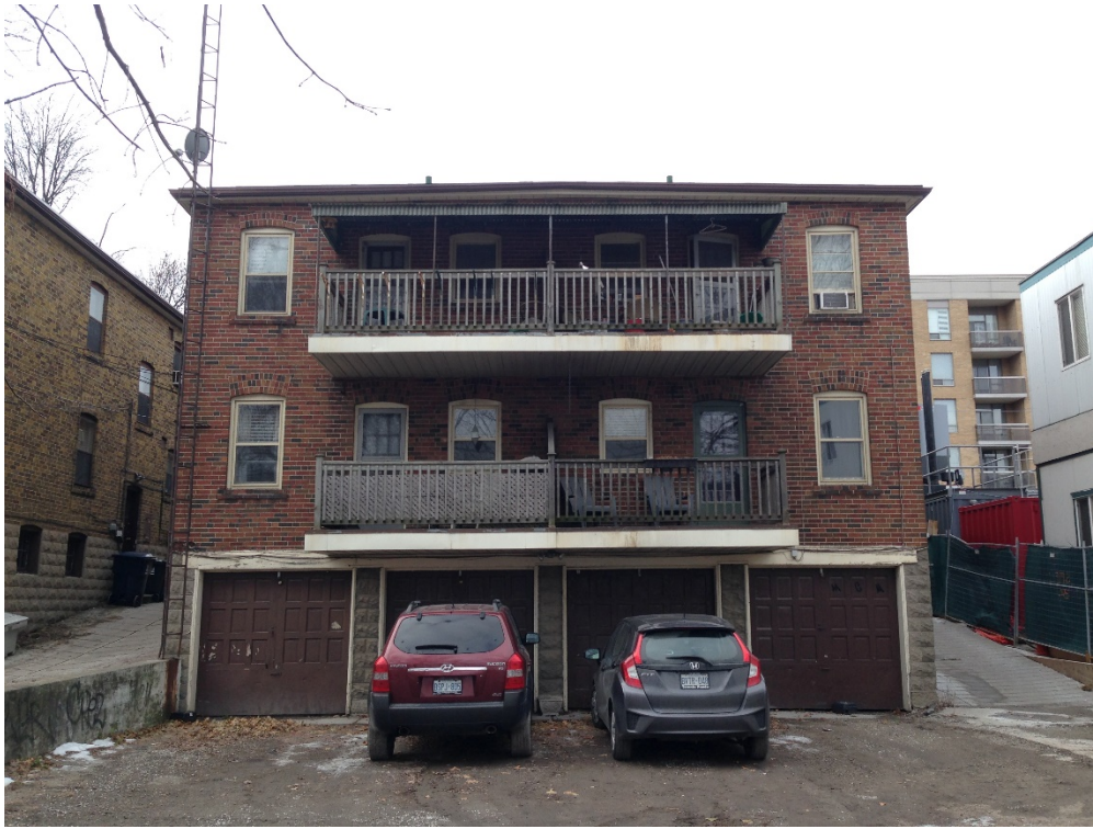
12. Rear (east) elevations of 1783-1785 Bayview Avenue showing the balconies and integrated garages. (HPS, 2017)
