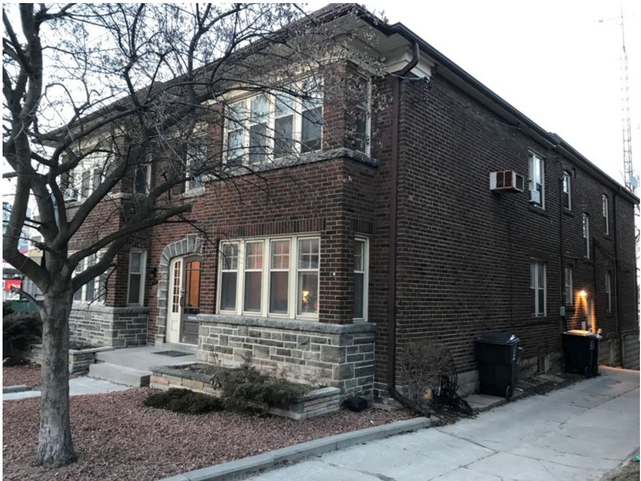
10. 1783-1785 Bayview Avenue, north and west elevations (HPS, 2018)
