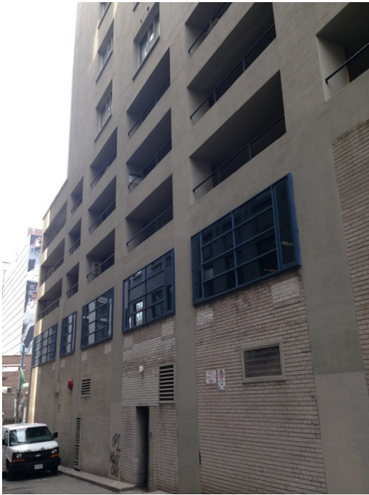
19. Carlton Tower, East elevation, showing the expressed concrete structure with the buff brick infill panels at grade and the continuation of the concrete wall surface on this east elevation of the office tower, and the post 1989 mezzanine level glazing patterns (HPS, 2018)
