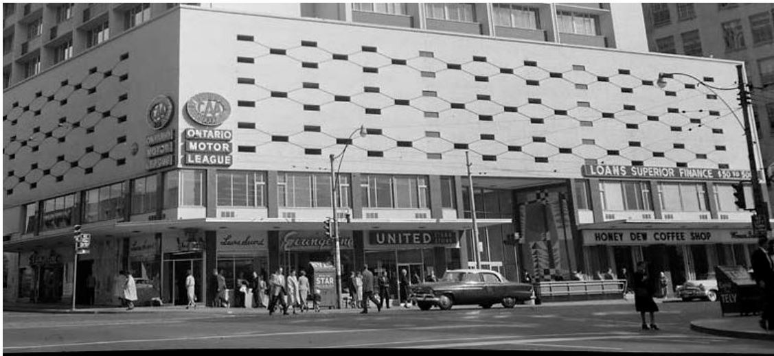
14. Detail of a 1960 photograph showing the podium with the original mullion patterns of the mezzanine glazing, the recessed double-height entrance with original artwork on the perpendicular wall and the entrance to the TTC subway just in front. CAA and the Ontario Motor League sign is prominently displayed. Note the original mezzanine window glazing pattern and that there are no skylights in the canopy. These were both altered in the 1989 renovations (CTA, Fonds 1257, F1257_s1057_it0727)
