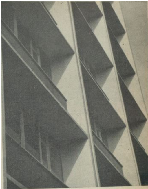
Above, a close-up of egg crate facade shows effectiveness of shading in mid-afternoon. Garage area (photo below is behind three storey with punched out window pattern. Main tower rises above.
