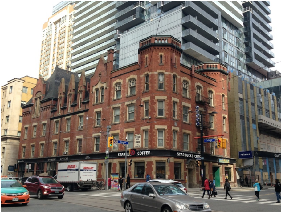
4. Oddfellows Building, 1892, north-west corner of College and Yonge streets (HPS, 2018)
