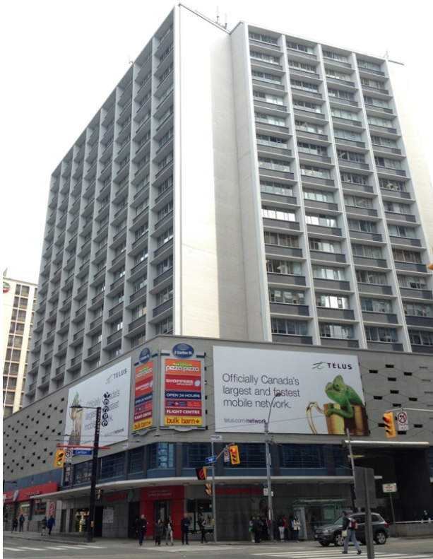
16. Carlton Tower, South and West elevations, viewed from the south on Yonge Street (HPS, 2018)
