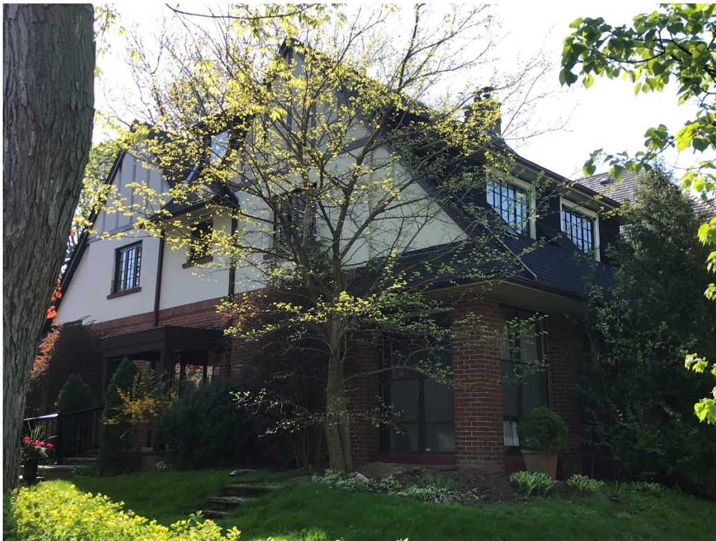
11. Albert E. Knox House, principal (north) and west elevations showing this corner lot as viewed from the intersection of Dinnick and Weybourne Crescents (HPS, 2018)
