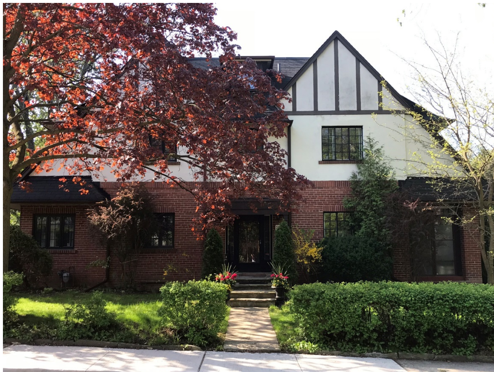
Above: Photograph of the principal (north) elevation at 35 Dinnick Crescent (Heritage Preservation Services [HPS], 2018) Cover: Photograph of the principal (north) elevation at 35 Dinnick Crescent (Google Street View, 2009)
