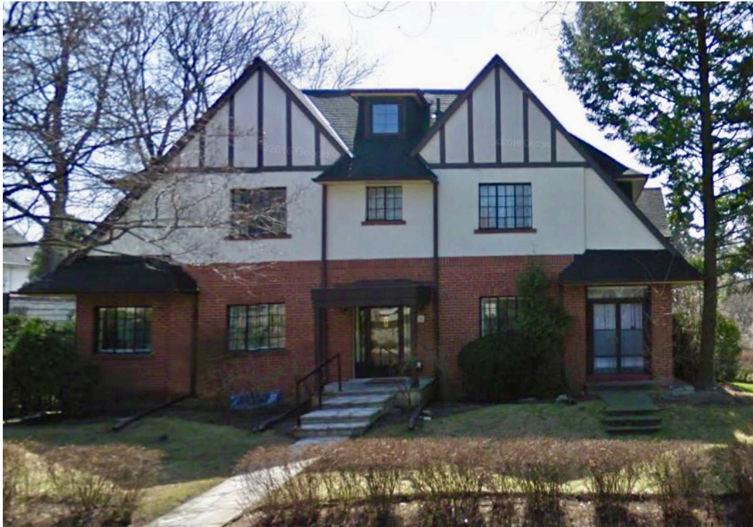
Photograph of the principal (north) elevation at 35 Dinnick Crescent (Google Street View, 2009)
