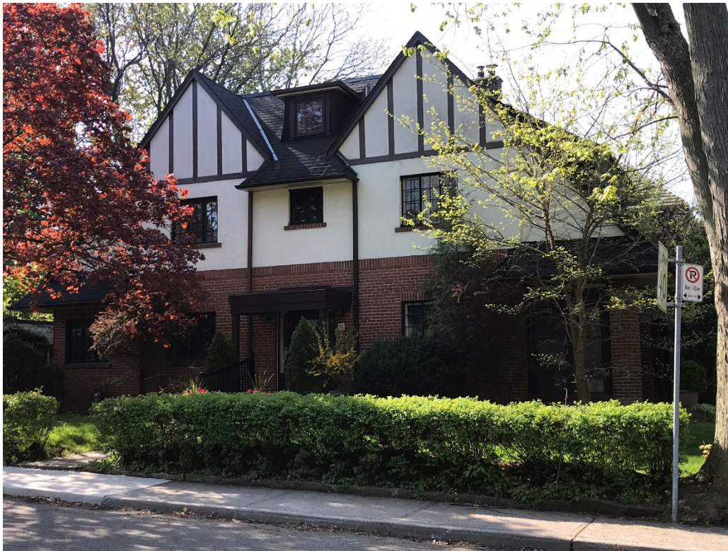
10. Albert E. Knox House, principal (north) elevation fronting Dinnick Crescent (HPS, 2018)
