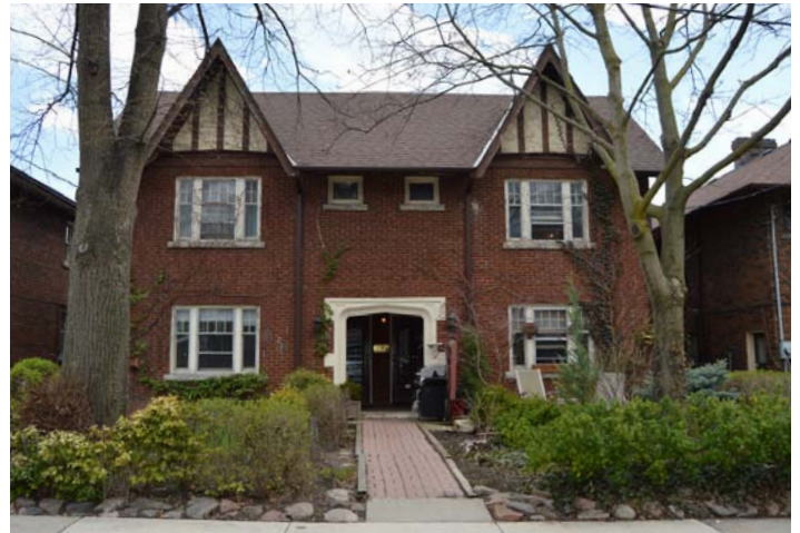
Figure 180: 21-23 Castle View Avenue
