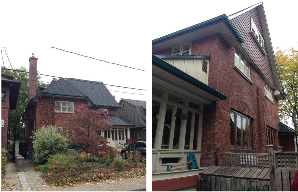
5a. principal (west) elevation (right) and north elevation (left); 5b. south elevation (right) showing the openings on the right where the two bay windows (shown on the drawings in Images 4a-4bb, above) were removed
