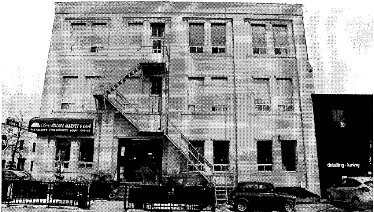
Figure 6: Photo of west facade of 65 Jefferson with a removable stucco finish on hard board insulation layer.
