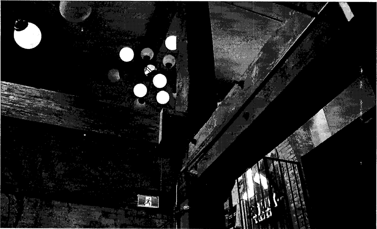
Figure 10: Exposed original post-and-beam framing at the Big Rock Brewery restaurant inside 60 Atlantic, accross Liberty Street from the Ontario Wind Engine and Pump Company Building.
