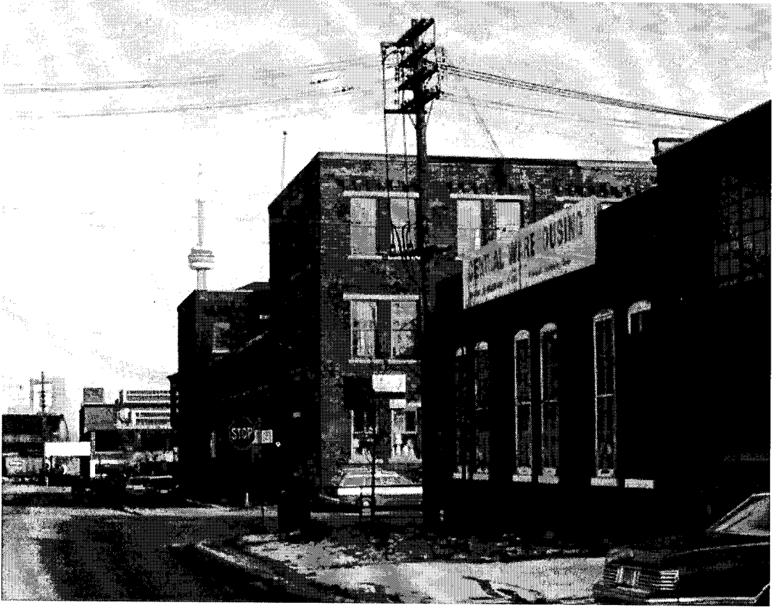
Figure 1: Photo looking east along Liberty Street at Jefferson Ave, c.1980s with all original brick facades intact on 35 Liberty and 65 Jefferson Ave.
