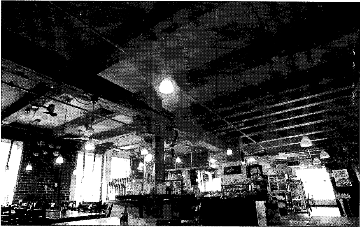
Figure 9: South view inside the ground floor of the Liberty Village Market and Cafe at 65 Jefferson Ave showing the exposed post-and-beam framing. This framing continues intact throughout the upper 2 floors of the building. The original post-and-beam framing is also intact throughout 35 Liberty Street.
