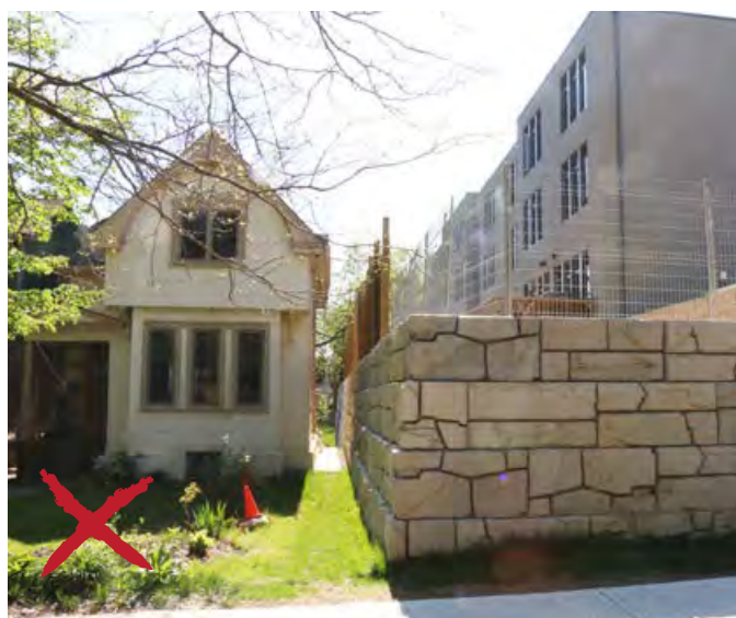
Grade alterations can create a negative impact on adjacent properties.
