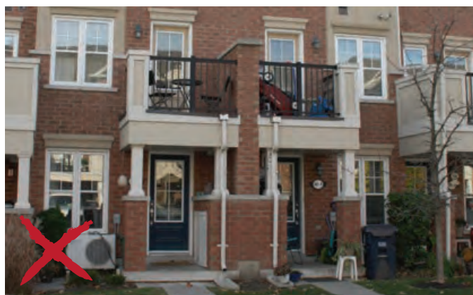
Example of a front facade over-cluttered with rainwater leaders, air conditioning units, utilities, and vents.
