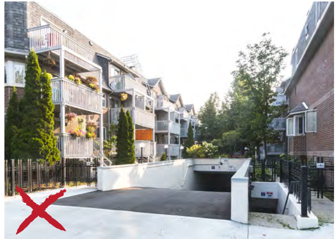
Avoid freestanding underground garage ramps and access stairs, incorporate within the building.
