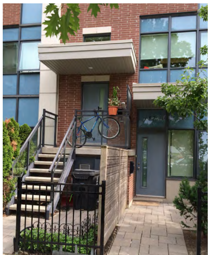
Accessible units at-grade are desirable in Stacked Townhouse building type. This project could be improved by internalizing some of the stairs to the upper units, a lighter canopy and more and better soft landscaping.
