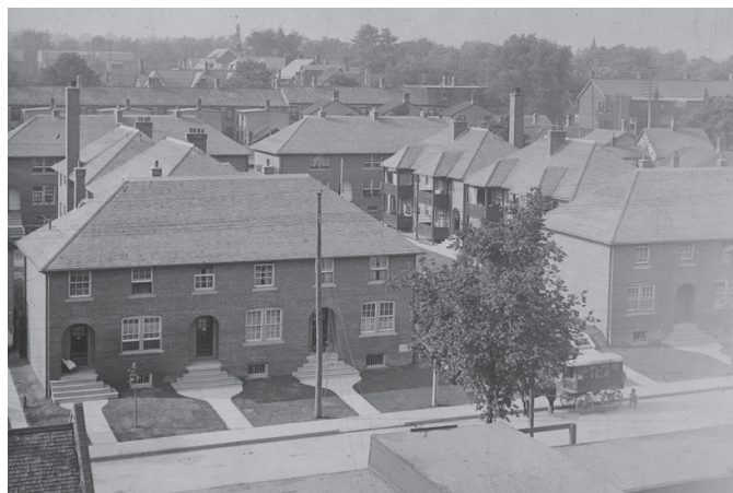
Spruce Court Apartments (completed in the 1920s), is one of the earliest examples of publicly supported, affordable, low-rise multi unit housing in Toronto. The 'Garden City' influence is prevalent through the use of large grassy, sunlit courtyards and play areas which were accessible to all units. Photo Credit: Spruce Court c1920, City of Toronto Archives, Fonds 1224.
