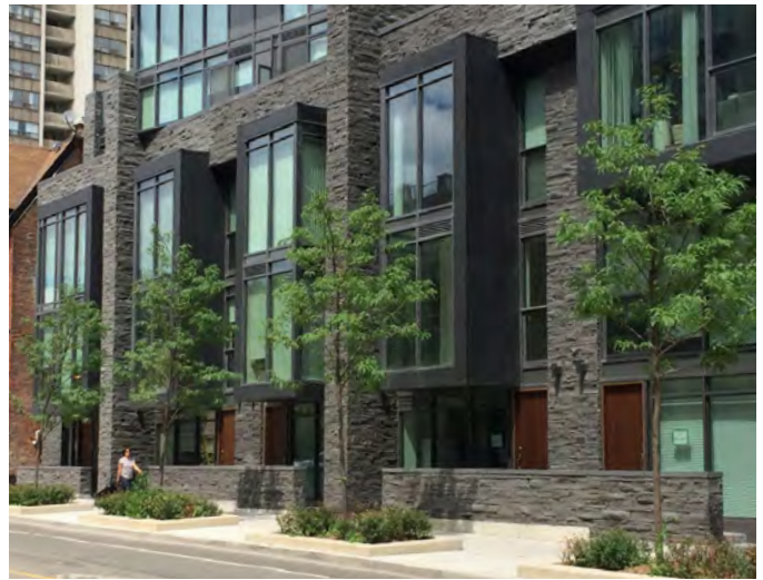
A new high-rise development incorporates townhouse units integrated into the base of the building.
