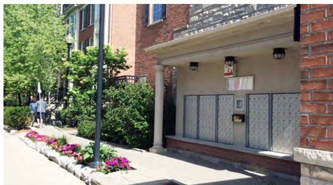
Good example of mail area integrated into building design with lighting and canopy.
