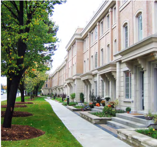
Good example of building relationship to grade with a minimal number of stairs. Existing trees have been preserved.
