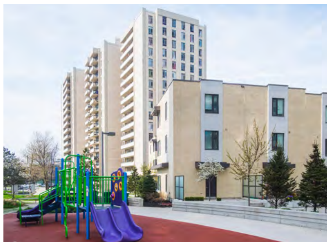
New low-rise development helps to improve existing negative site conditions and create new shared amenity areas for all residents.
