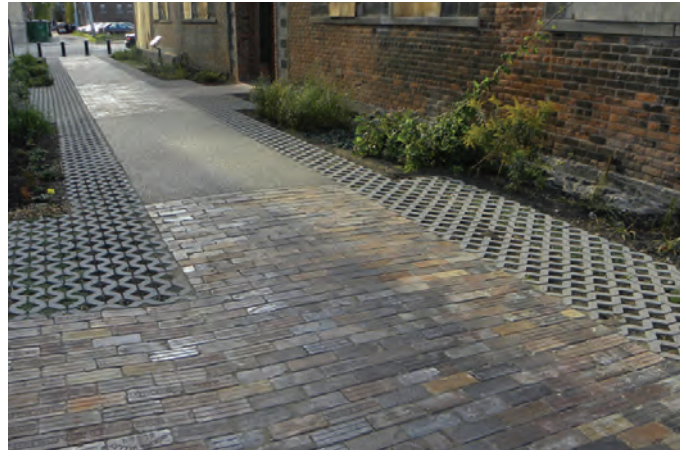
Permeable paving allows for water infiltration. Credit: National Association of City Transportation Officials.
