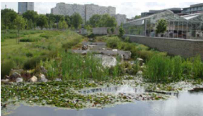
Valleys, ponds and large sunken surfaces collect and treat rainwater, run off and floodwater from the Seine River, Saint Ouen, France
