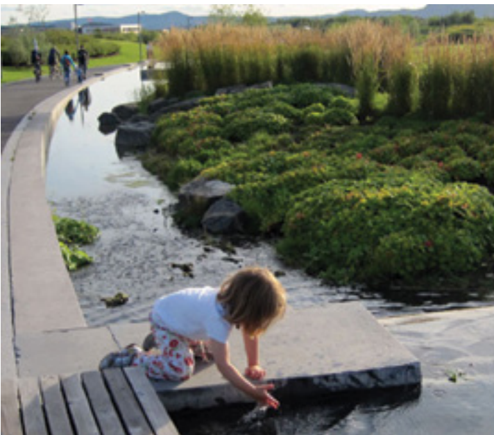
Nansen Park is designed to receive surface water from adjacent housing areas and roads with open green swales to carry water to the nearby lake, and biological sand filters, mechanical filters and pumps to clean and aerate the water, Oslo, Norway
