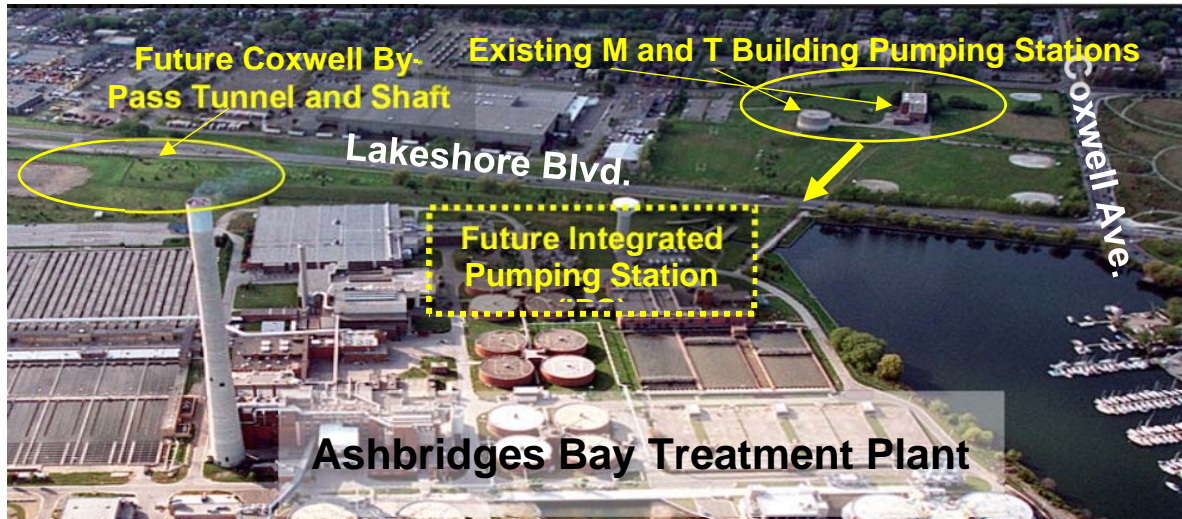
Figure 1. Aerial view showing existing M and T Building Pumping Stations, future Integrated Pumping Station, and the future Coxwell By-Pass Tunnel shaft location north of the ABTP.
