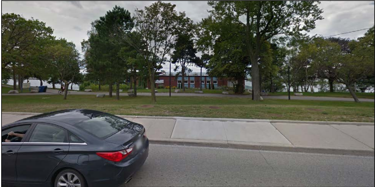
North Elevation of Building viewed from Lake Shore Boulevard West
