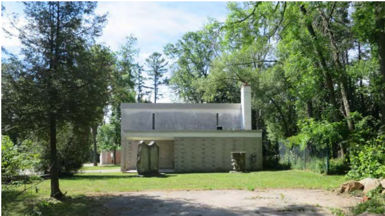
View of the north (side) elevation of Building 191 at 201 Guildwood Parkway, looking south (HIA July 2017 - revised May 2018, Taylor Hazell Architects Ltd.).
