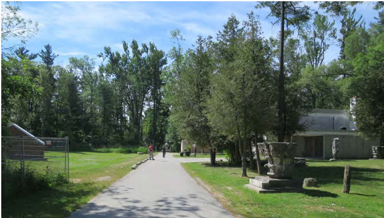
Contextual view of Building 191 at 201 Guildwood Parkway, looking south and showing the north (side) elevation (HIA July 2017 - revised May 2018, Taylor Hazell Architects Ltd.).
