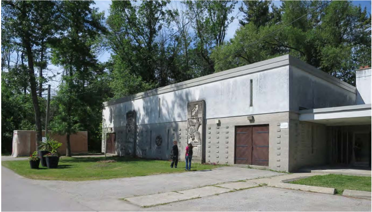
View of the east (front) elevation of Building 191 at 201 Guildwood Parkway, looking southwest (HIA July 2017 - revised May 2018, Taylor Hazell Architects Ltd.).
