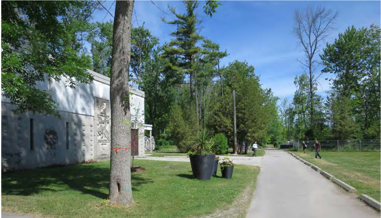
View of the east (front) elevation of Building 191 at 201 Guildwood Parkway, looking north (HIA July 2017 - revised May 2018, Taylor Hazell Architects Ltd.).
