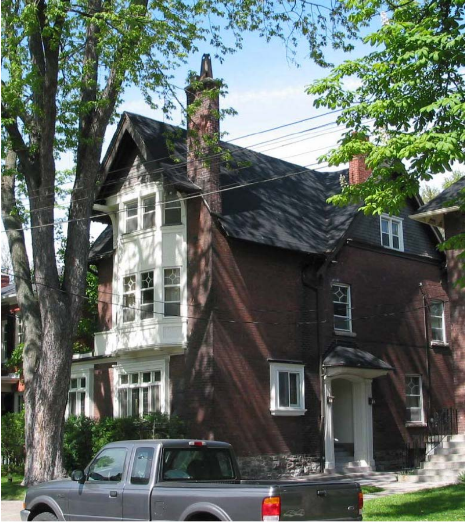
33 Sherbourne Street North- view from street looking northeast
