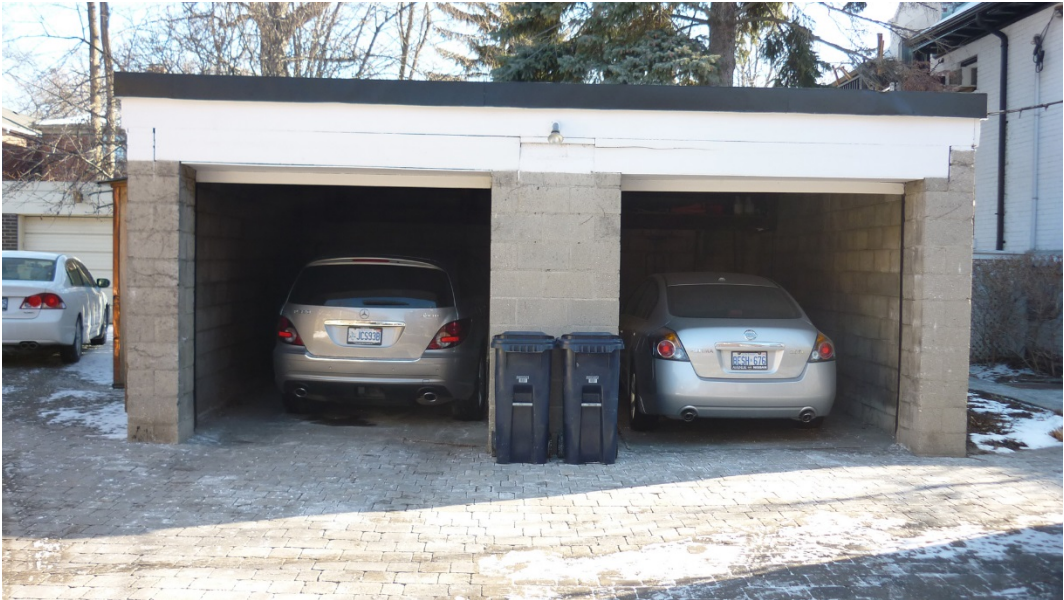
Typical garage- a total of five of these structures will be demolished
