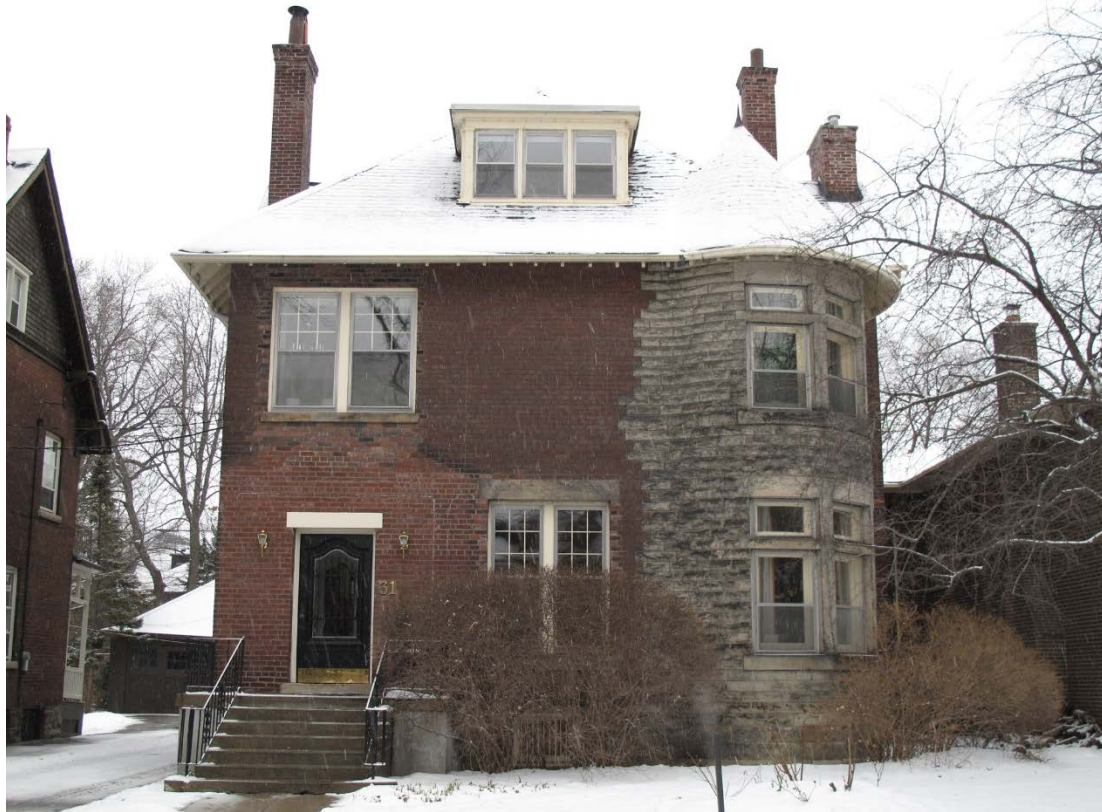
33 Sherbourne Street North- "C" Category building
