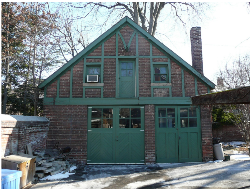
Coach house located at rear of 31 Sherbourne St. N.
