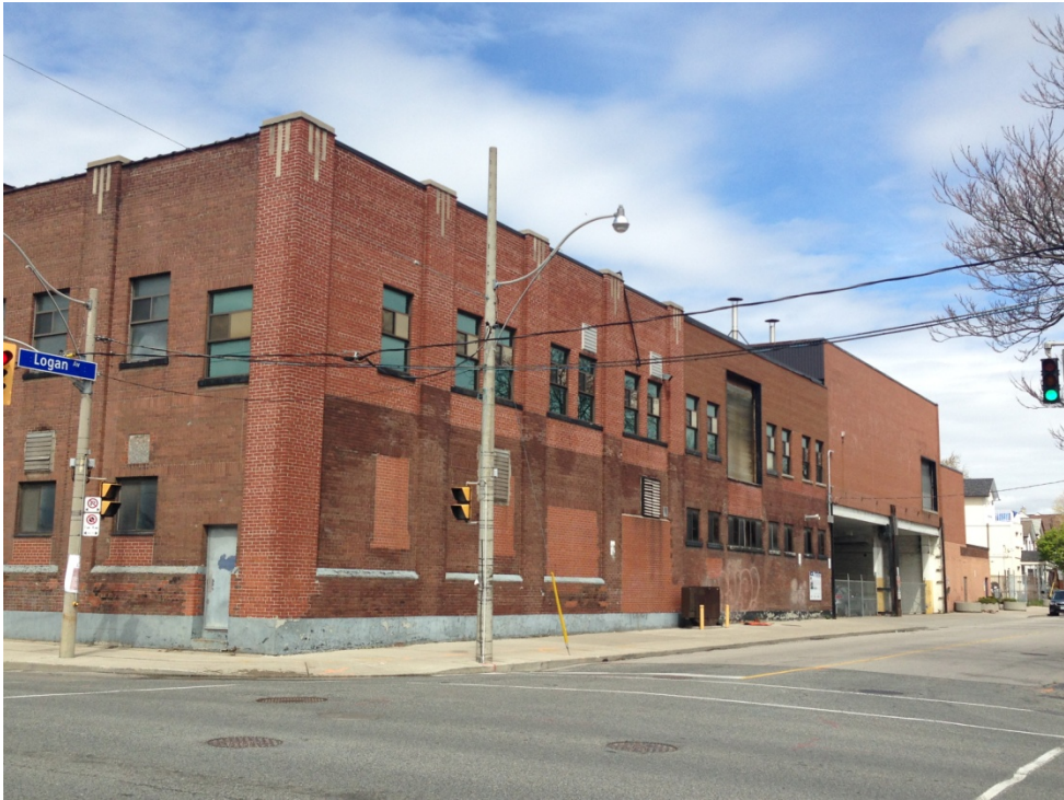
462 Eastern Avenue: Looking Northwest, Showing the South and East Elevations
