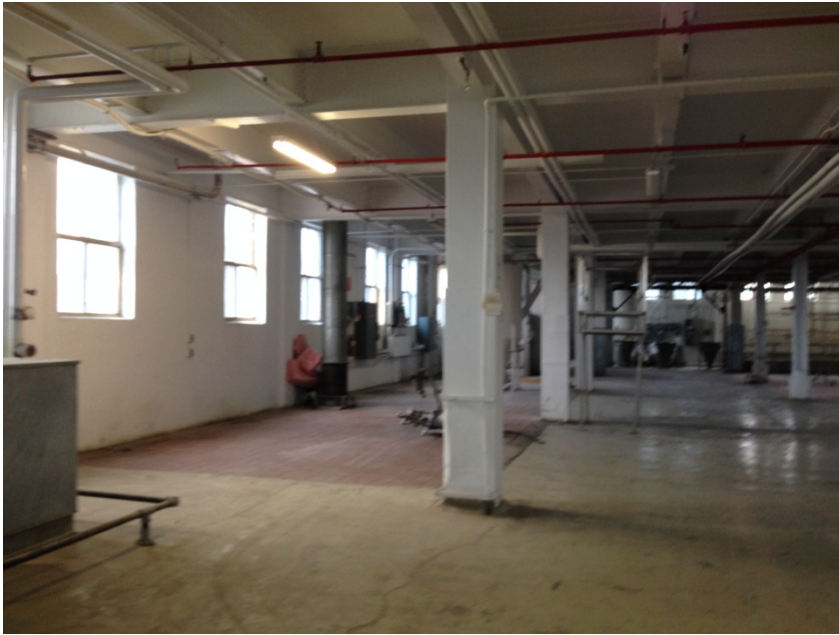
17. Interior of the 1926 building, fourth floor showing internal structure
