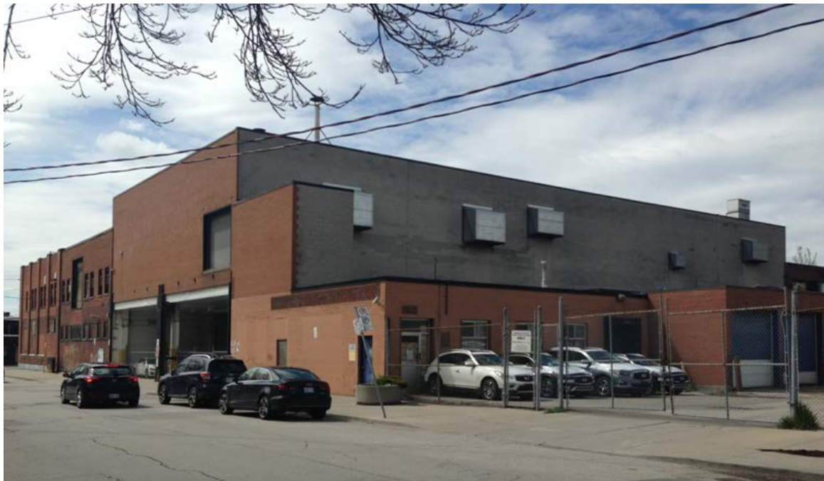
25. Side and north elevations as seen from Logan Avenue (HPS, 2017)
