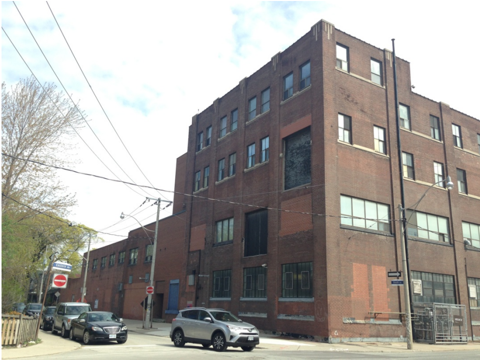
462 Eastern Avenue: Looking Northeast, Showing the West and South Elevations
