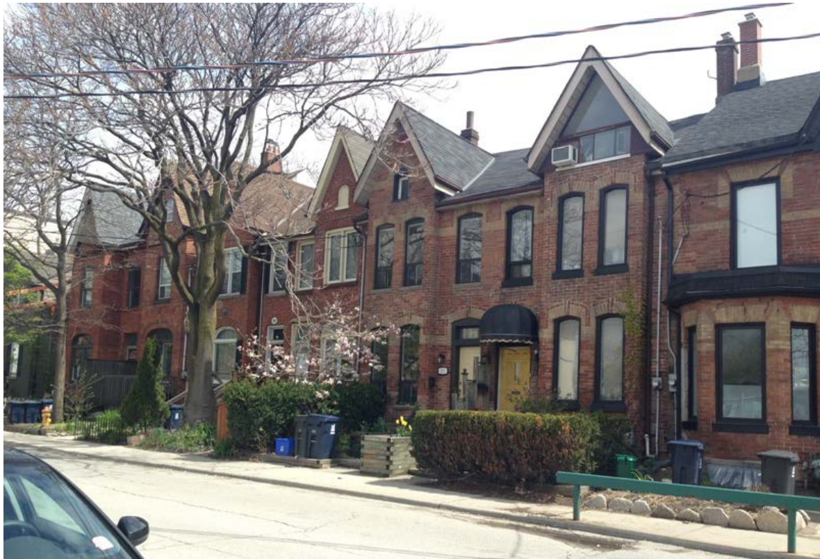
33. Logan Avenue, east side, north of Eastern Avenue, opposite Brown's Bread Ltd. (HPS, 2017)
