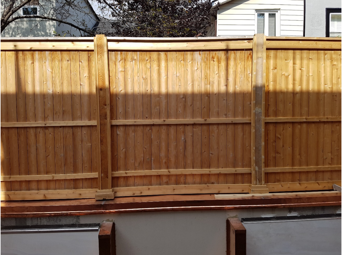
Photo of rear yard 36 Berryman St.
