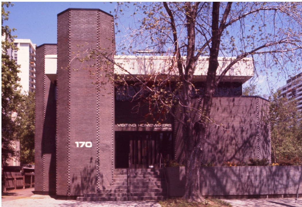
Early photograph of the VHA building showing the original pigment of the concrete brick cladding and paving (Leslie Rebanks)
