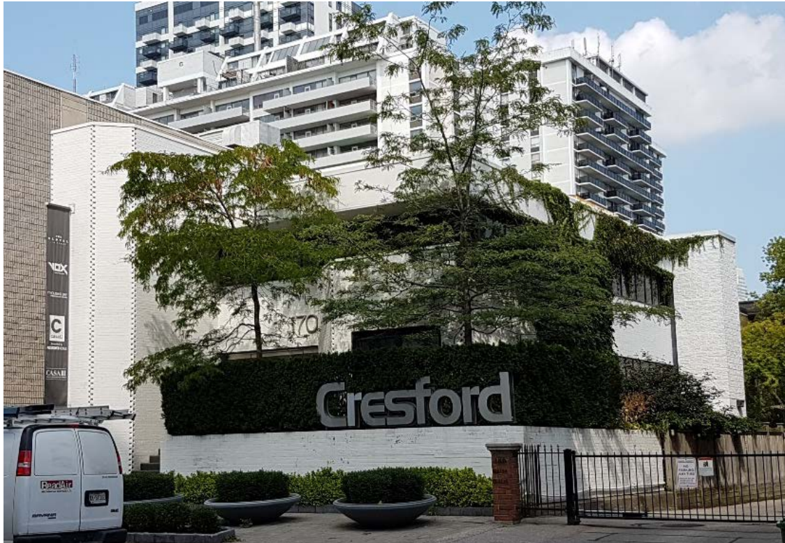
Photograph of the VHA building, principal (south) and side (east) elevations (HPS, 2017)
