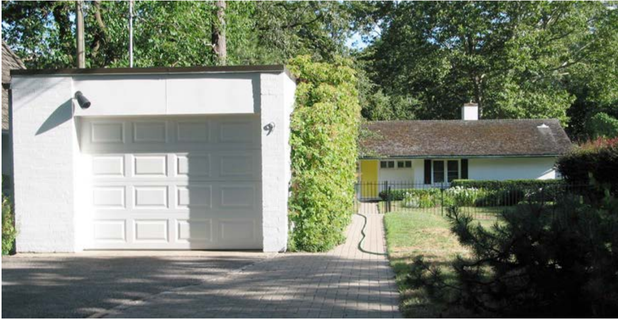
9 Dale Avenue- north view of property garage structure to left with house beyond
