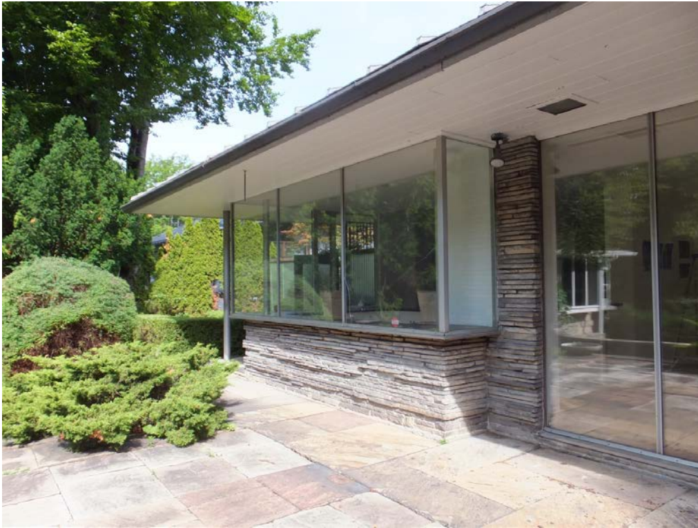
7 Dale Avenue- view of partial south elevation
