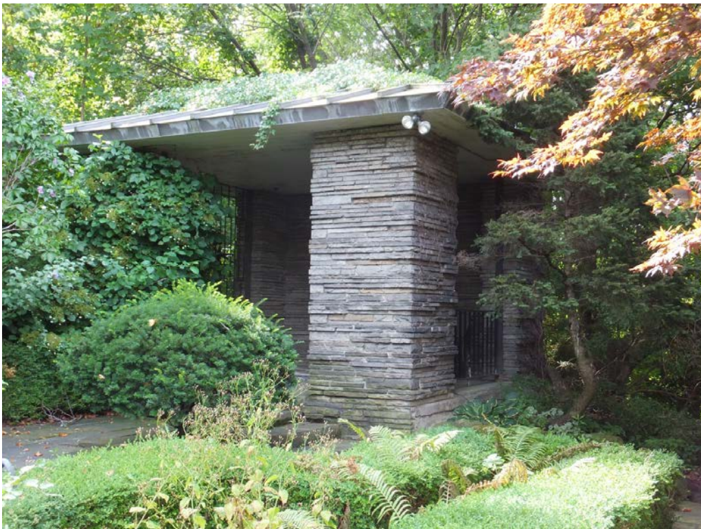
7 Dale Avenue- teahouse structure in rear yard
