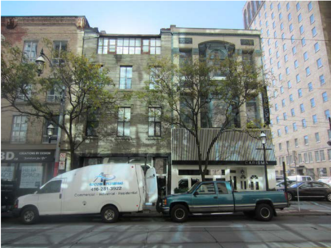
King Street East elevations of 71, 75 and 79 King Street East.
