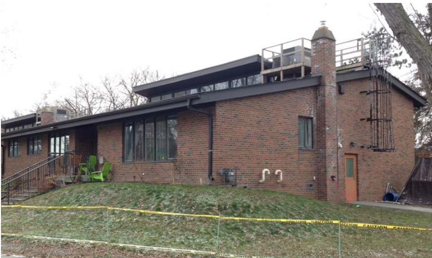
20. West (Side) and North (Principal) elevation of a typical cottage. (HPS, 2017)
