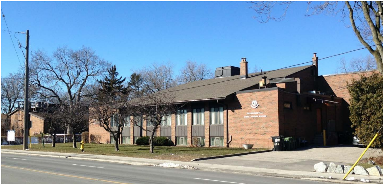
Photograph of the Salvation Army Broadview Village, with the Margaret R. and Harry A. Newman Building (right), principal (east) elevation, and one of the cottages on the far left showing a side (east) elevation (HPS, 2018)
