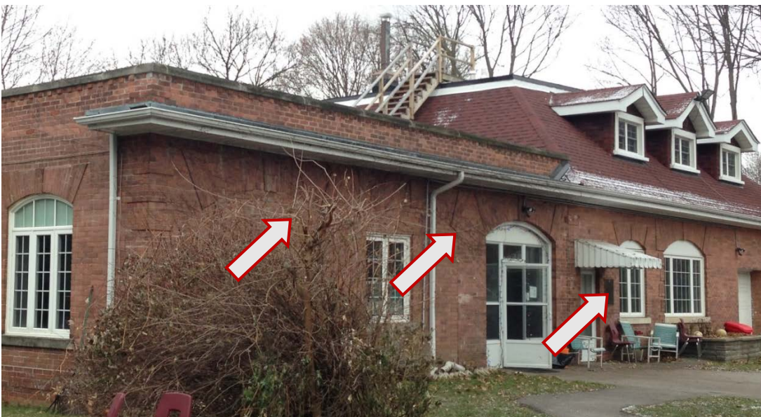
12. West and East Elevation, Coach House. The arrows indicate the brick arches and voussoirs which remain following the 1961 brick infills. Next to the canopy the quins indicate the edge of the original coach house before the south wings was added (HPS, 2017)
