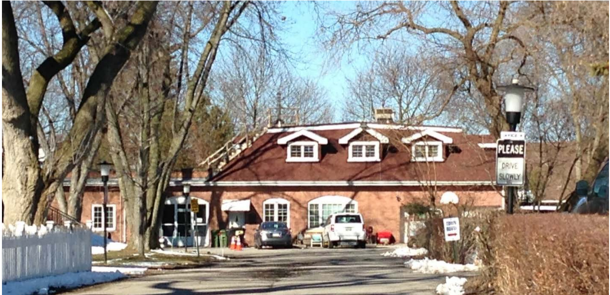
Photograph of the Taylor-Davies family Chester Park Coach House principal (east) elevation as viewed along the driveway from Broadview Avenue. (Heritage Preservation Services [HPS], 2018)
