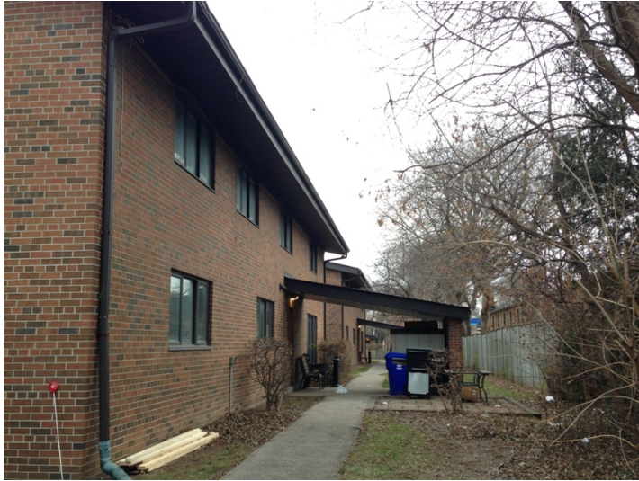
21. South (Rear) elevation of a typical cottage showing the bicycle shed. (HPS, 2017)
