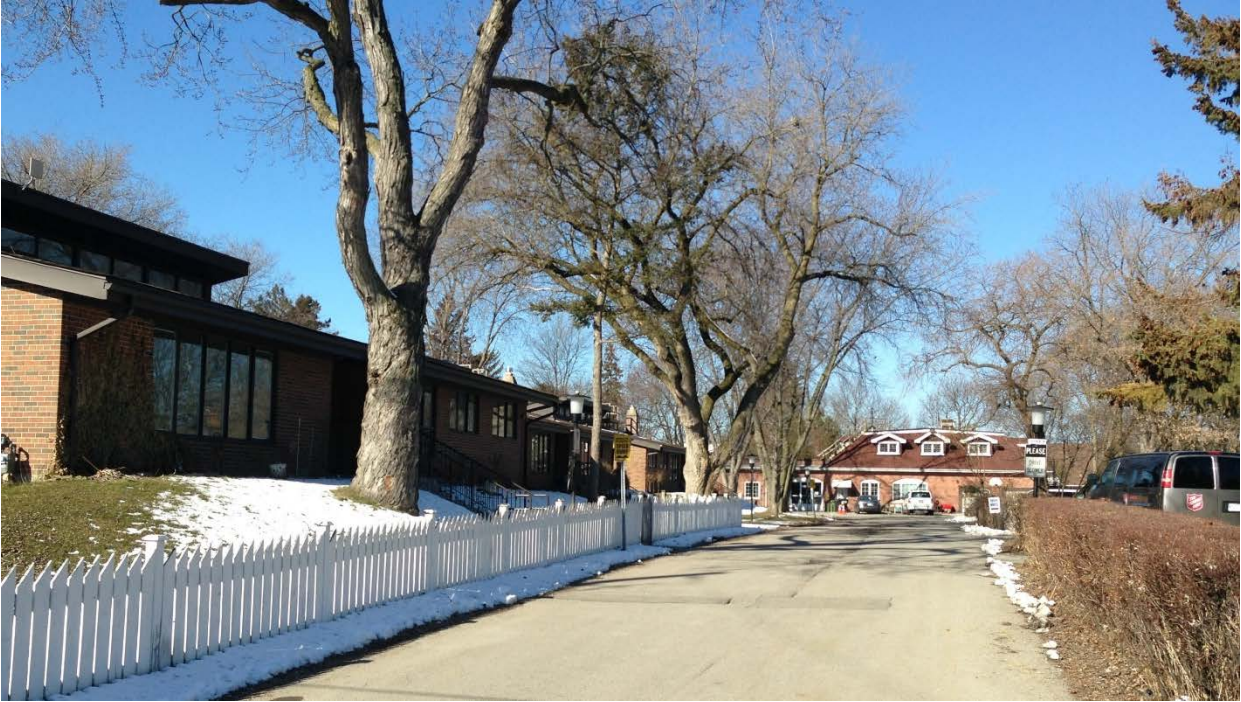
Above: View from Broadview Avenue down the driveway past the three "cottages" to the Chester Park coach house (Heritage Preservation Services [HPS], 2018) Cover: Salvation Army Broadview Village, Margaret R. Newman and Harry A. Newman Administrative Building and the side elevation of one of the cottages (HPS, 2018)
