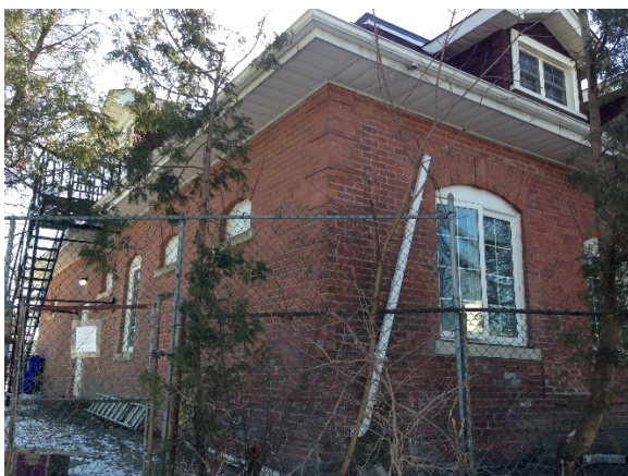
15. West and North Elevation of the Coach House showing the windows and the brick detail (HPS, 2018)
