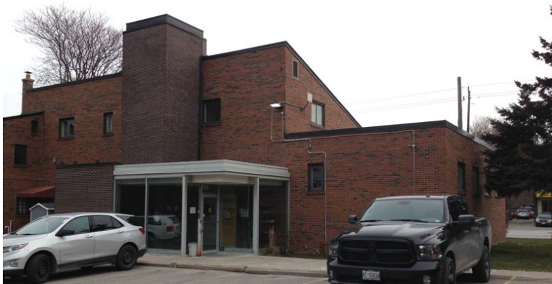
29-32. Photographs showing the principal east and side (south) elevations, the Salvation Army insignia above the building's name acknowledging the Newman's (top), the rear west elevation (middle) and the new entry and elevator addition (2010) (below) (HPS, 2017-2018)
