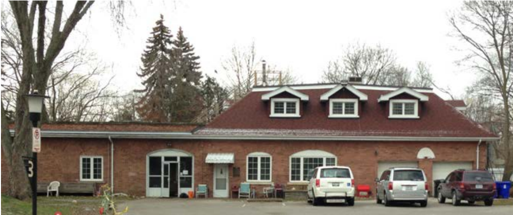
10. East Elevation of the Coach House (HPS, 2017)
