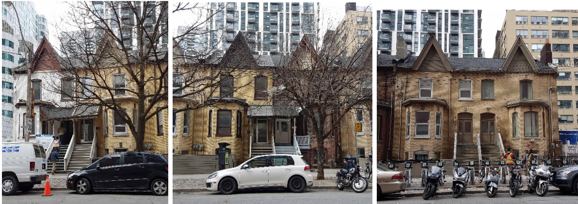
4a.-4c. principal (east) elevations of the Widmer Street Row Houses at 10-12 Widmer (left), 14-16 Widmer (centre), and 18-20 Widmer (right)
