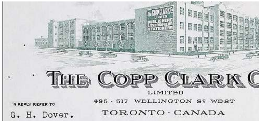
4e. Illustration, Copp Clark Company Complex, 1940
