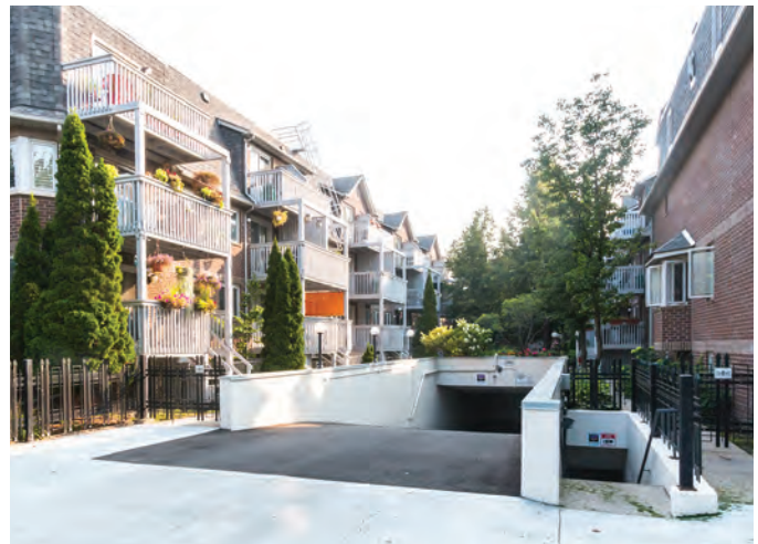
Avoid freestanding underground garage ramps and access stairs, but rather incorporate these within the building.
