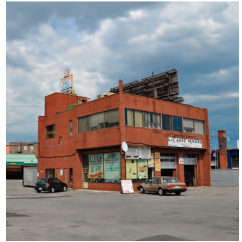
Auto-related uses such as auto body shops, car wash, gas station occupy most of the area in the Dundas Point Precinct. This area has large paved surfaces with very little greenery.
