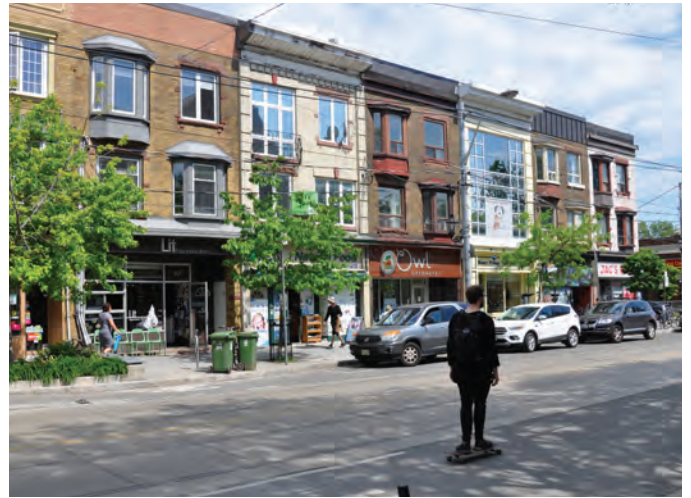
Roncesvalles Main Street Precinct - Typical three-storey mixed use buildings.
