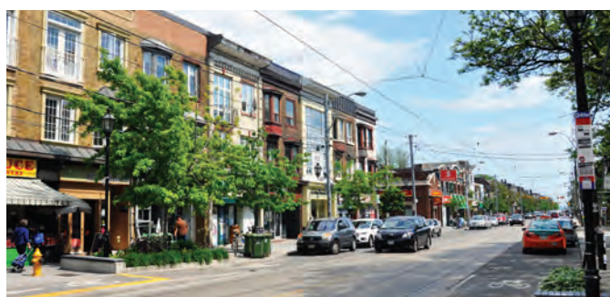
A relatively consistent 'street wall' along Roncesvalles Avenue with predominately two to three-storey buildings lining the street. The street is mostly a 'main street' in character with a rich mix of retail and commercial uses.
