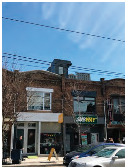
A stair access addition to a two-storey building.
