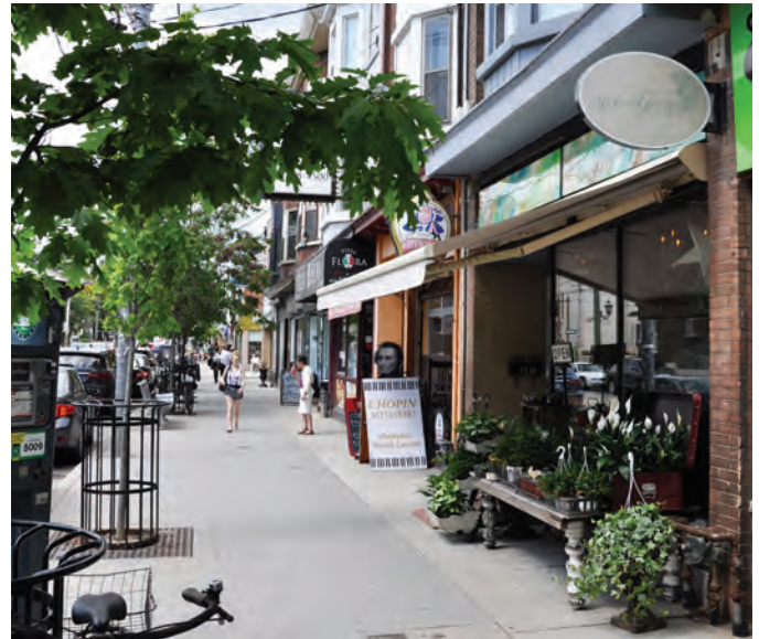
Solid building materials combined with fine-grained retail create an attractive streetscape. With access and loading activities at the rear of properties, the primary street frontage can be uninterrupted by service activities.
