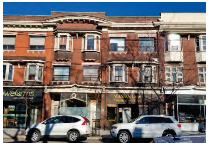
Example of a Commercial Block with Residential Accommodation Above at 99, 101, 103, 105 Roncesvalles Avenue.
