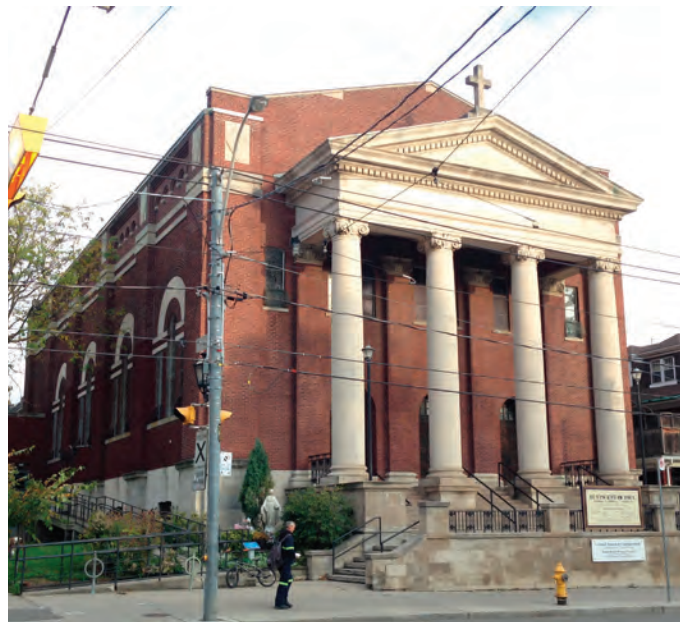
Example of a Landmark Community Building at 265 Roncesvalles Avenue.
