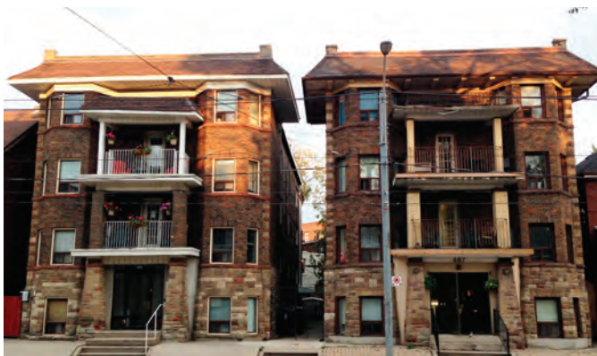
Example of a Low-rise Apartment Block at 467, 469 Roncesvalles Avenue.
