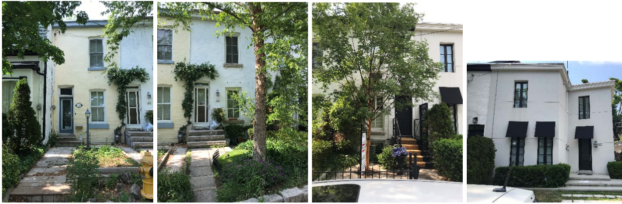
9. (From left to right) The principal (south) elevations of 116, 118, 120 and 122 Shaftesbury Avenue, respectively (HPS, 2018).
