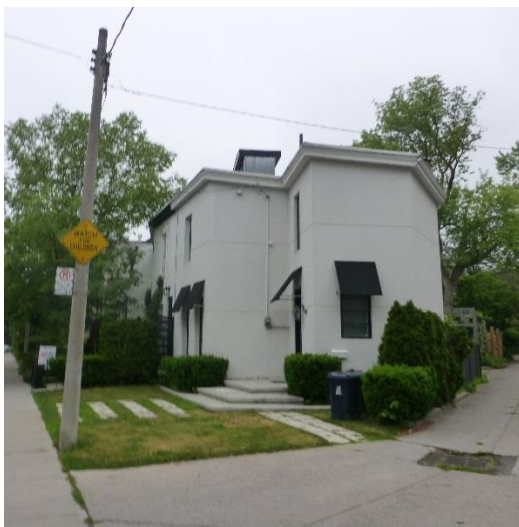
122 Shaftesbury and Street/Lane Intersection
