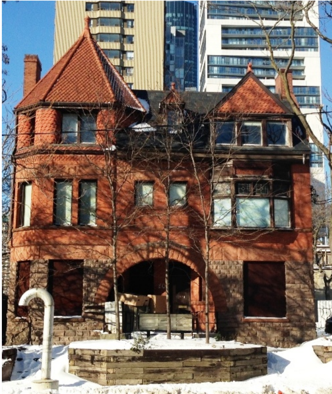
Photograph of the listed heritage property at 280 Jarvis Street with semi-detached houses showing the principal (east) elevation. (Heritage Preservation Services, March 2019)
