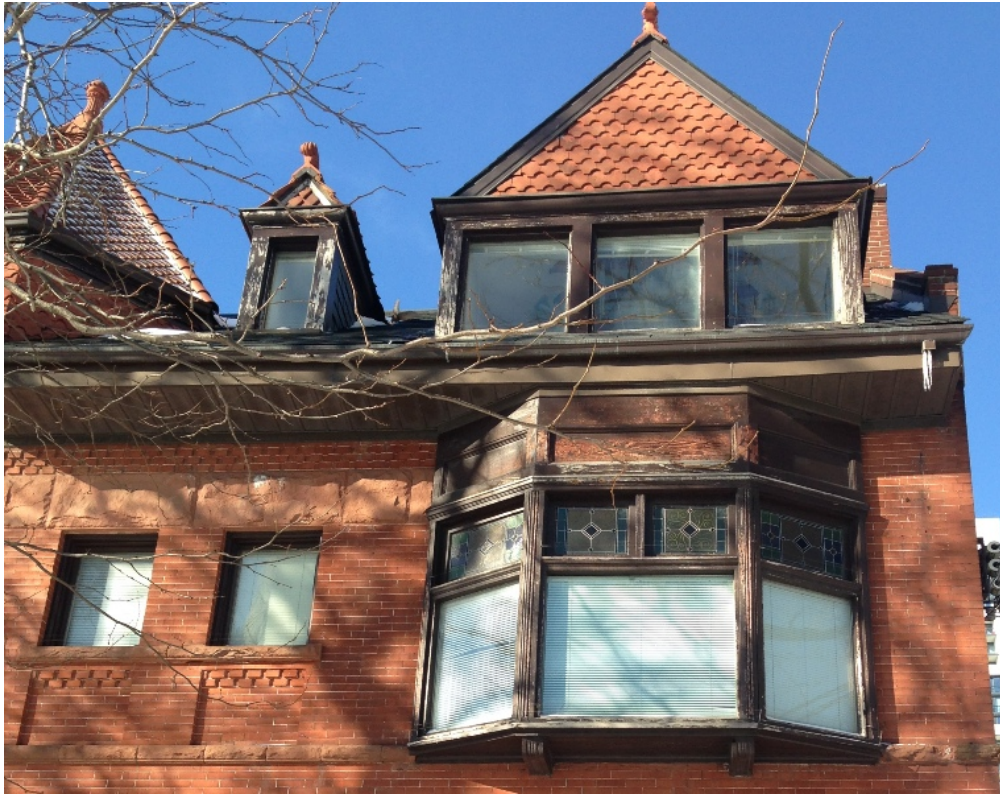
29. 280 Jarvis Street, showing the detailing on the north half of the principal (east) elevation with the bay window with stained glass, panels, mouldings and brackets, the terracotta finials on the roof dormers, the combination of scalloped and diamond shaped tiles in the dormer and the surface texture created by the brick patterns and relief and the rusticated sandstone blocks. (HPS, 2019)
