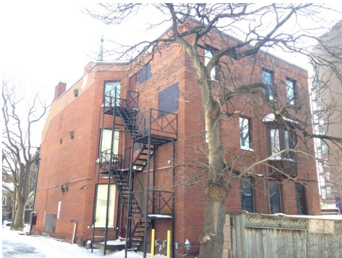
30. 280 Jarvis Street, showing the side (north) and rear (east) elevations. The rear wing has acquired a third floor addition, but otherwise retains the original building foot print (HPS, 2019)
