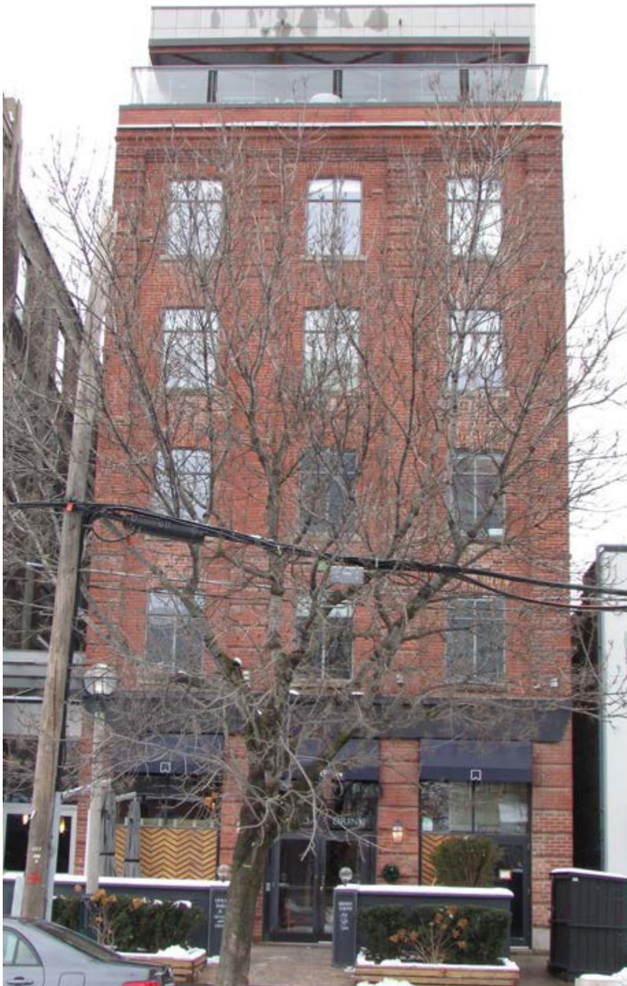
482 Wellington Street West – South/primary façade. Note 1998 rooftop addition.
