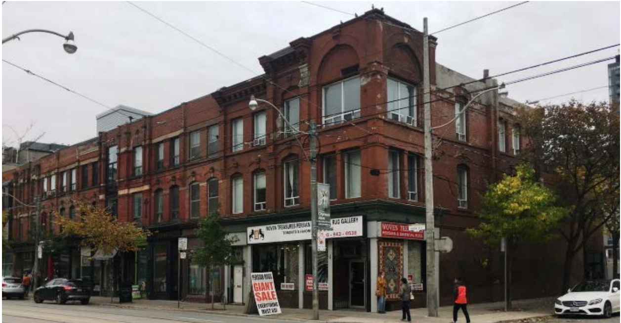
167-185 Queen Street East, photograph of the block showing the principal (north) elevation facing Queen Street East and side (west) elevation facing George Street. (Heritage Planning [HP] 2019)
