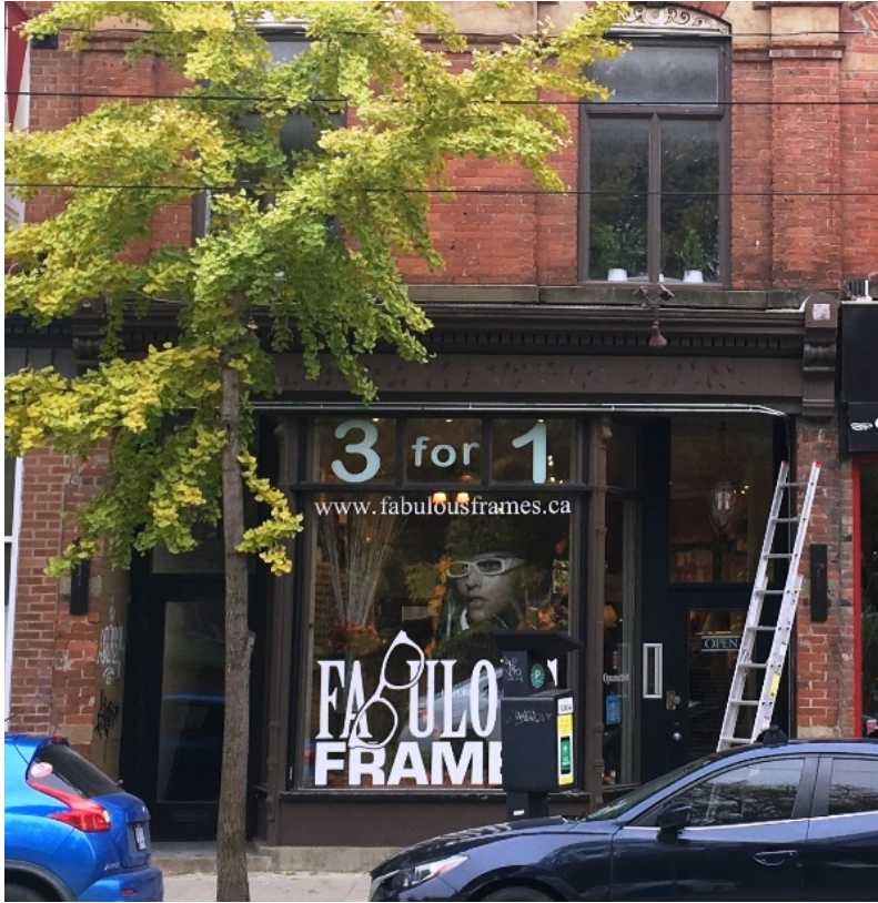
22. 185 Queen Street East, shopfront showing the original pattern of the two recessed entrances with the bay window, its decorative colonettes and the cornice and entablature above. (HP, 2019)
