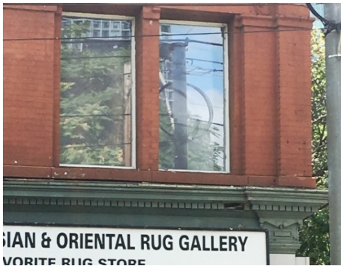
19. 167 Queen Street East, detail of the wood cornice above the shopfront (HP, 2019)
