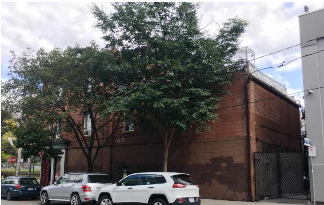
23. 167 Queen Street East, side (west) elevation facing George Street showing the 1968 rear addition (HP, 2019)
