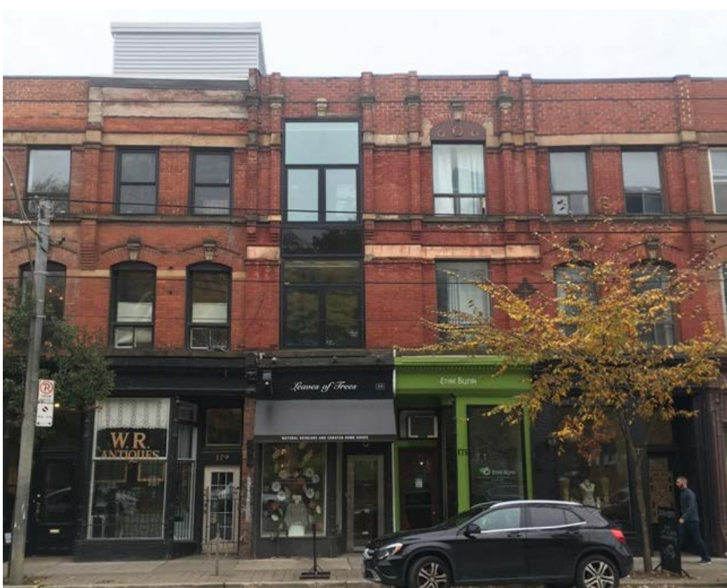
17. Photograph of the properties at 173, 175, 177 and 179 Queen Street East showing the principal (north) elevations (HP, 2019)
