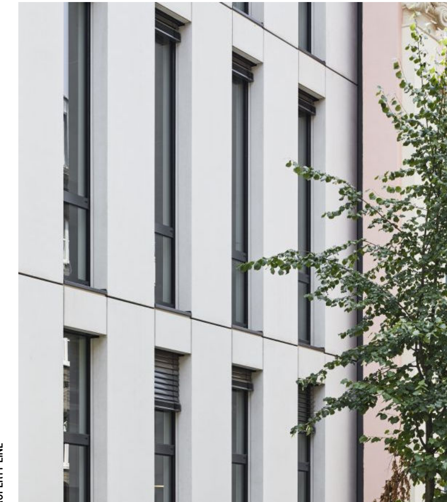
Precedent Images of Precast masonry panel and glazing
