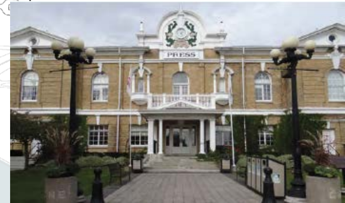
The Press Building, 2018
