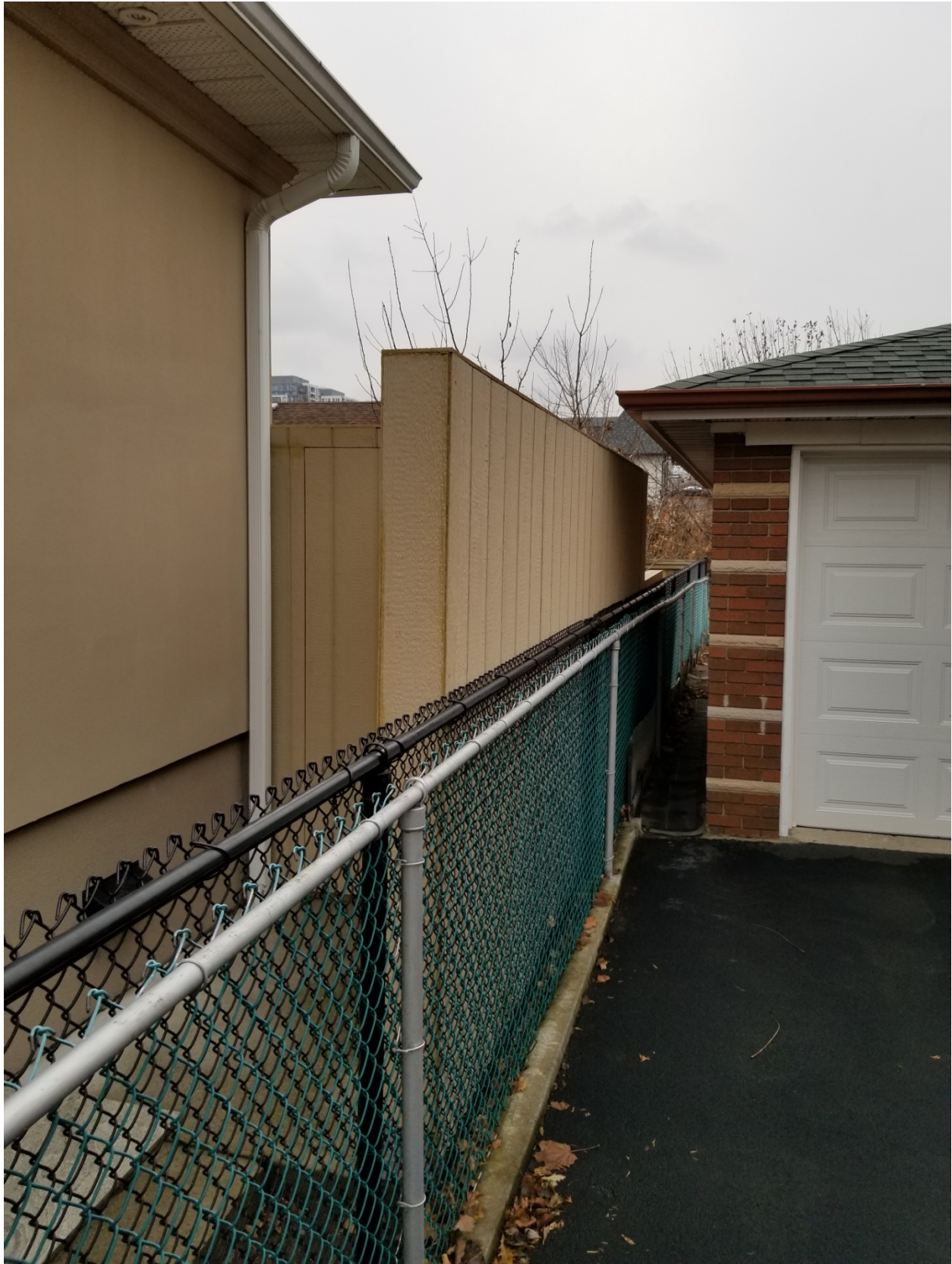
Attachment 4: West facing view from 916 Islington Ave towards 914 Islington Ave
