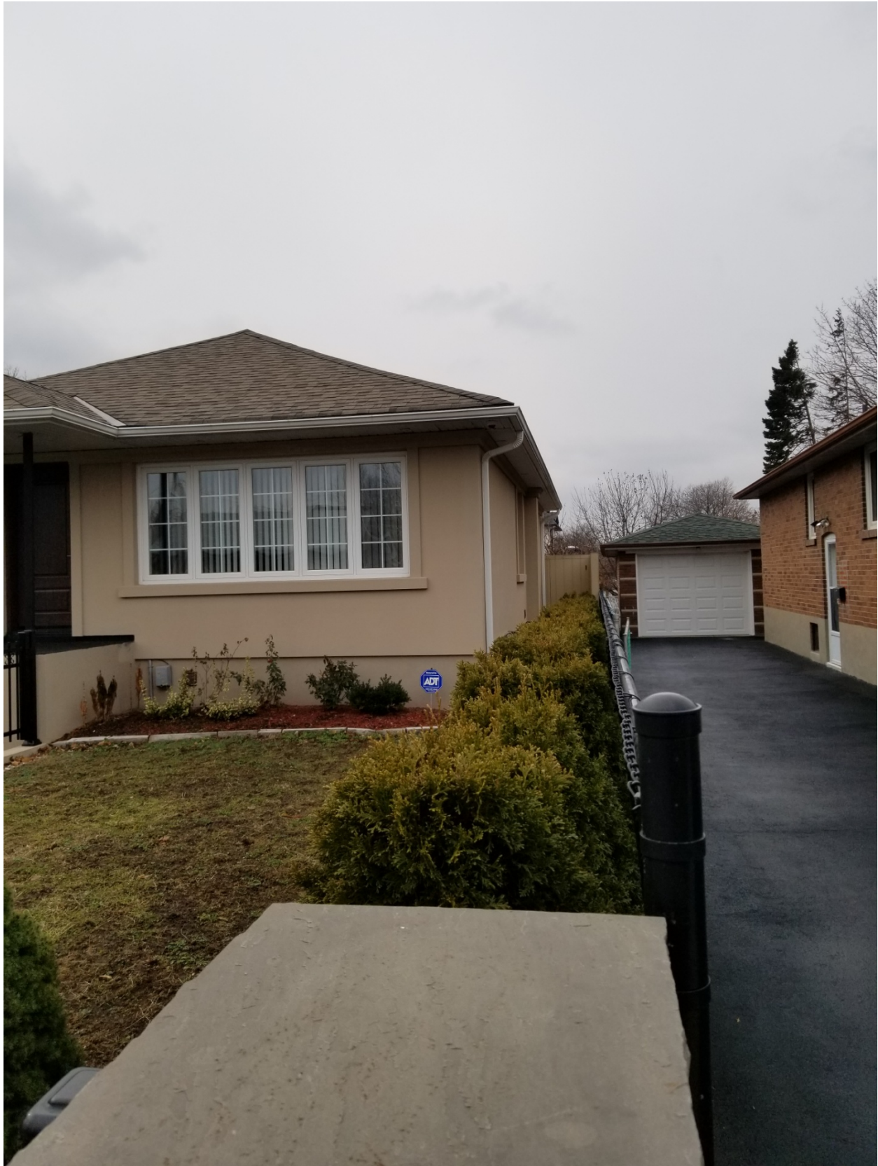
Attachment 3: West facing view from Islington between 914 / 916 Islington Ave
