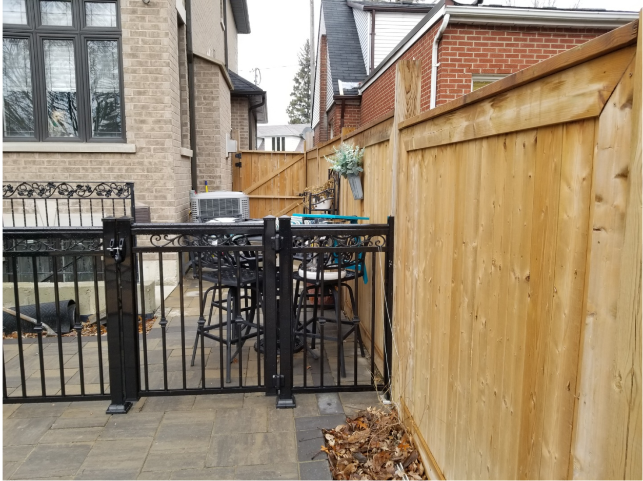
Attachment 7: North facing view of pool enclosure and gate
