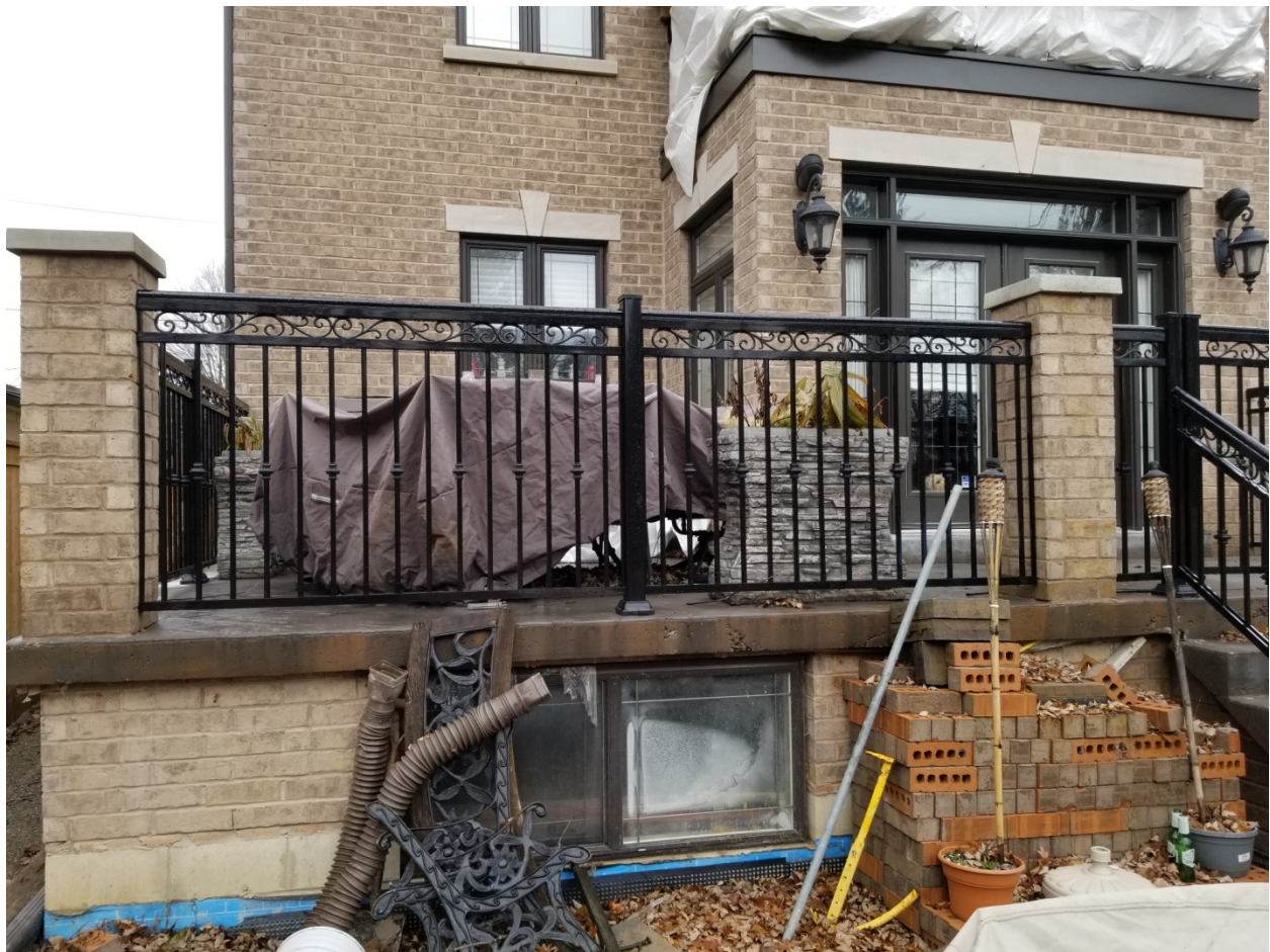
Attachment 4: North facing view of dwelling walkout patio with pool enclosure
