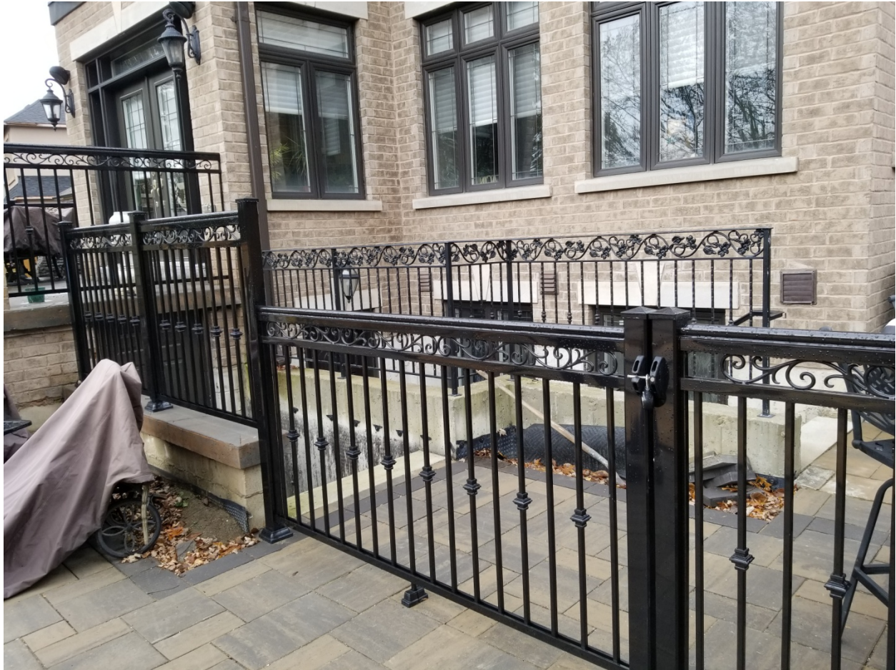
Attachment 6: North facing view of pool enclosure and gate
