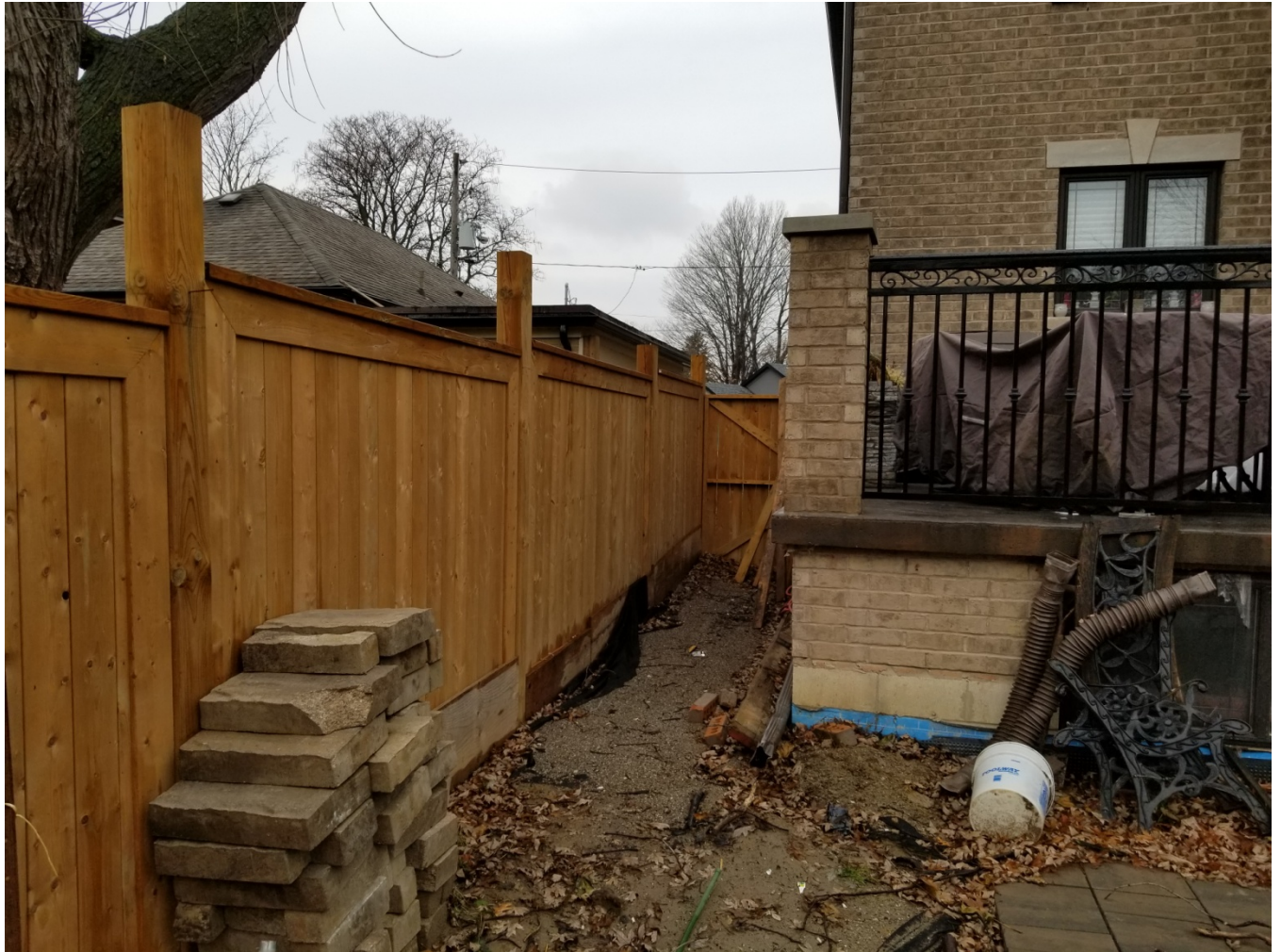
Attachment 3: North facing view exterior fence and patio pool enclosure
