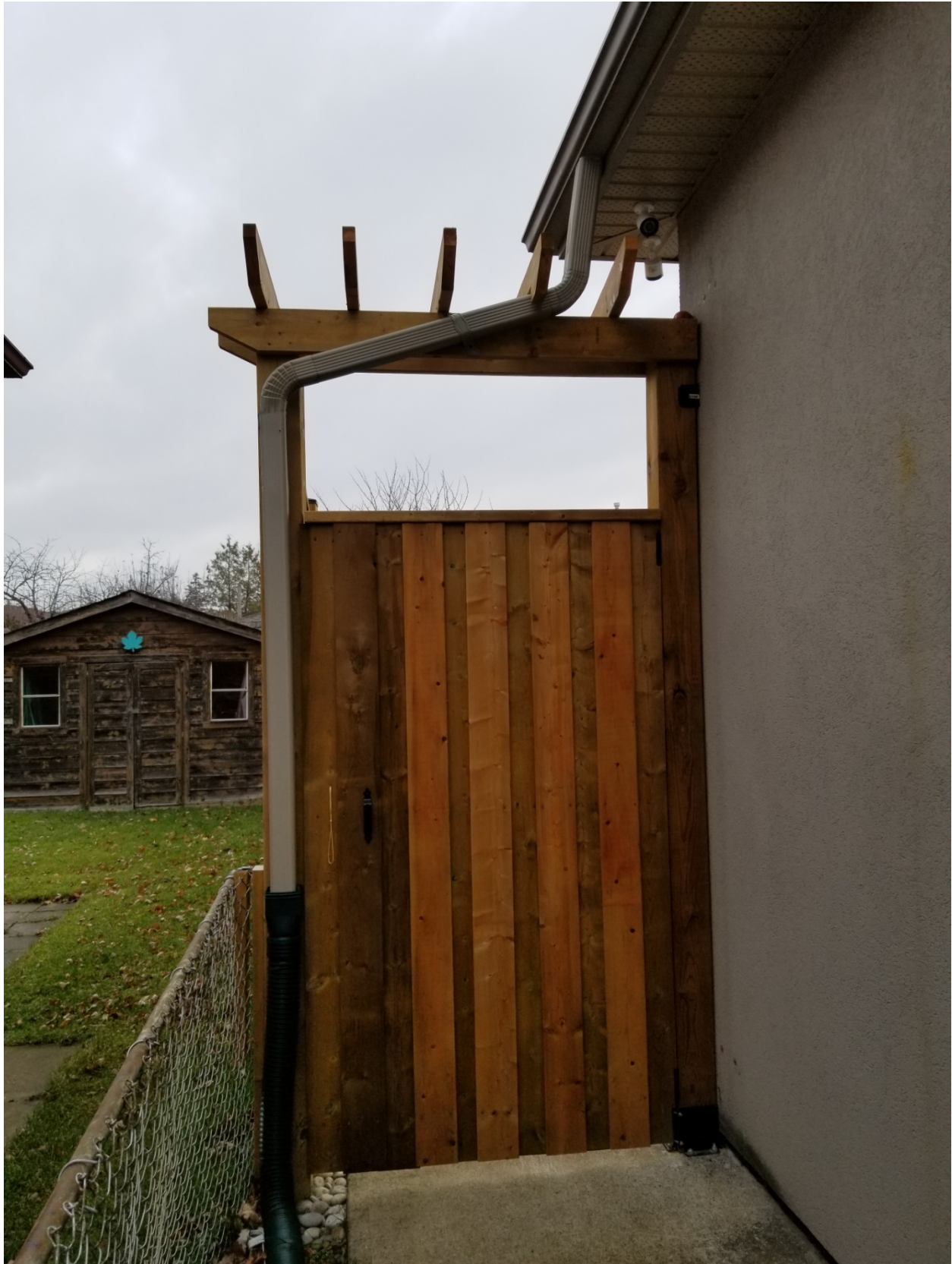
Attachment 3: East facing view from side of property towards rear yard
