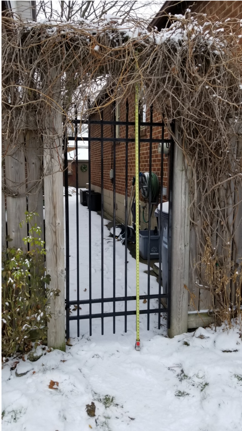
Attachment 3: West facing view from side yard of 60 Parker Ave
