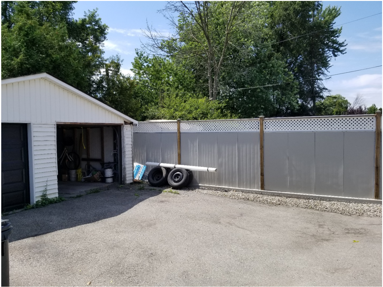
Attachment 2: Rear Yard Fence of 184 Royal York Road, South West exposure
