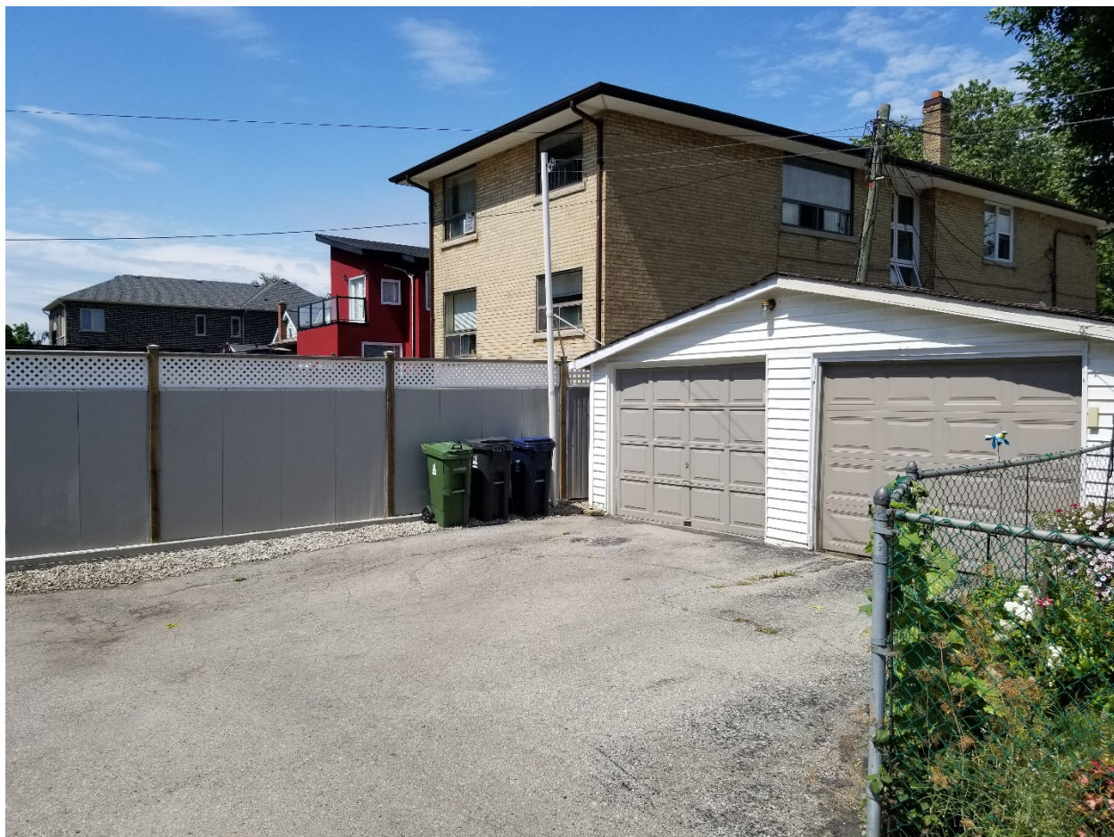
Attachment 2: Rear Yard Fence of 190 Royal York Road, South West exposure
