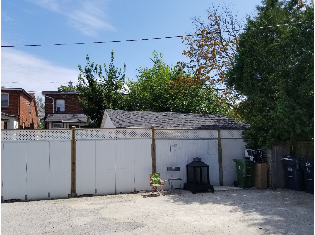
Attachment 3: Rear Yard Fence of 186 Royal York Road, South West Exposure
