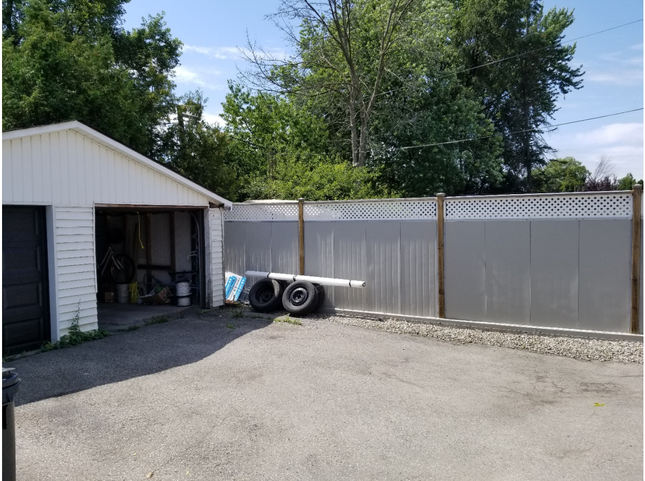
Attachment 2: Rear Yard Fence of 186 Royal York Road, South West exposure
