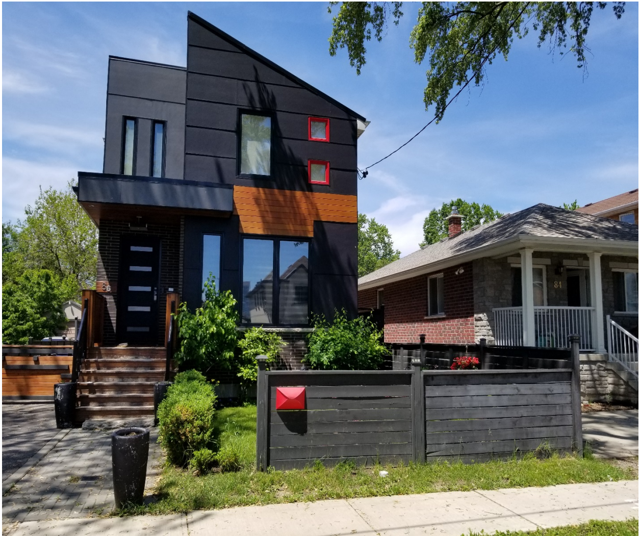
Attachment 4: Front Yard Fence of 86 Waniska Ave, Northern Exposure
