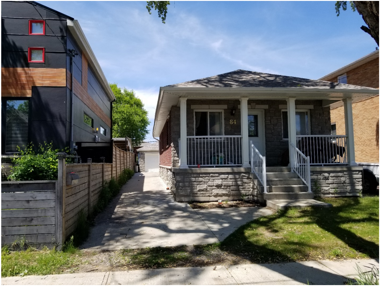
Attachment 2: Front Yard Fence of 84 Waniska Ave, Northern exposure
