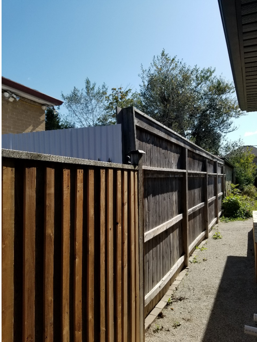
Attachment 3: Rear Yard Fence of 373 Rustic Road
