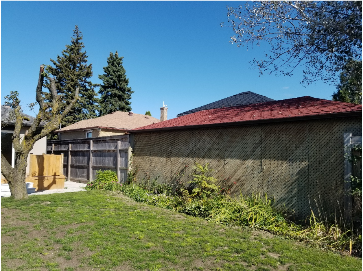
Attachment 2: Rear Yard Fence of 373 Rustic Road from 371 Rustic Road
