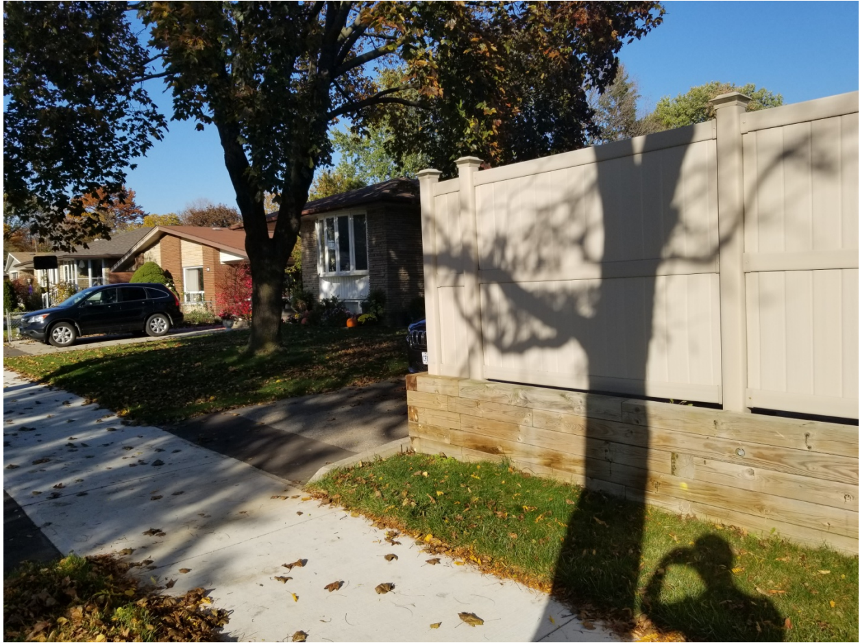
Attachment 3: Rear Yard Fence of 54 Harrop Ave facing Northbound
