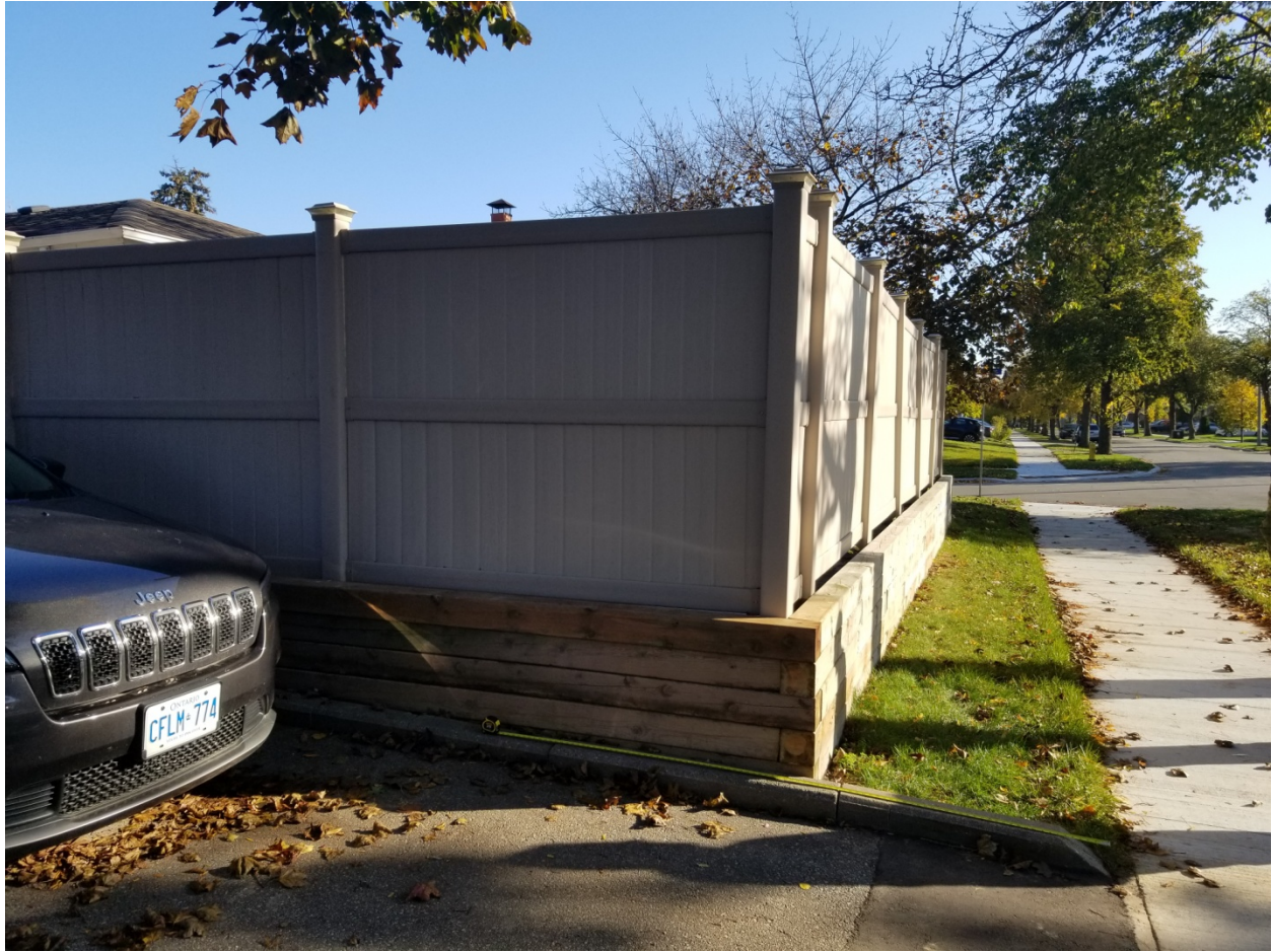
Attachment 2: Rear Yard fence facing South towards 54 Harrop
