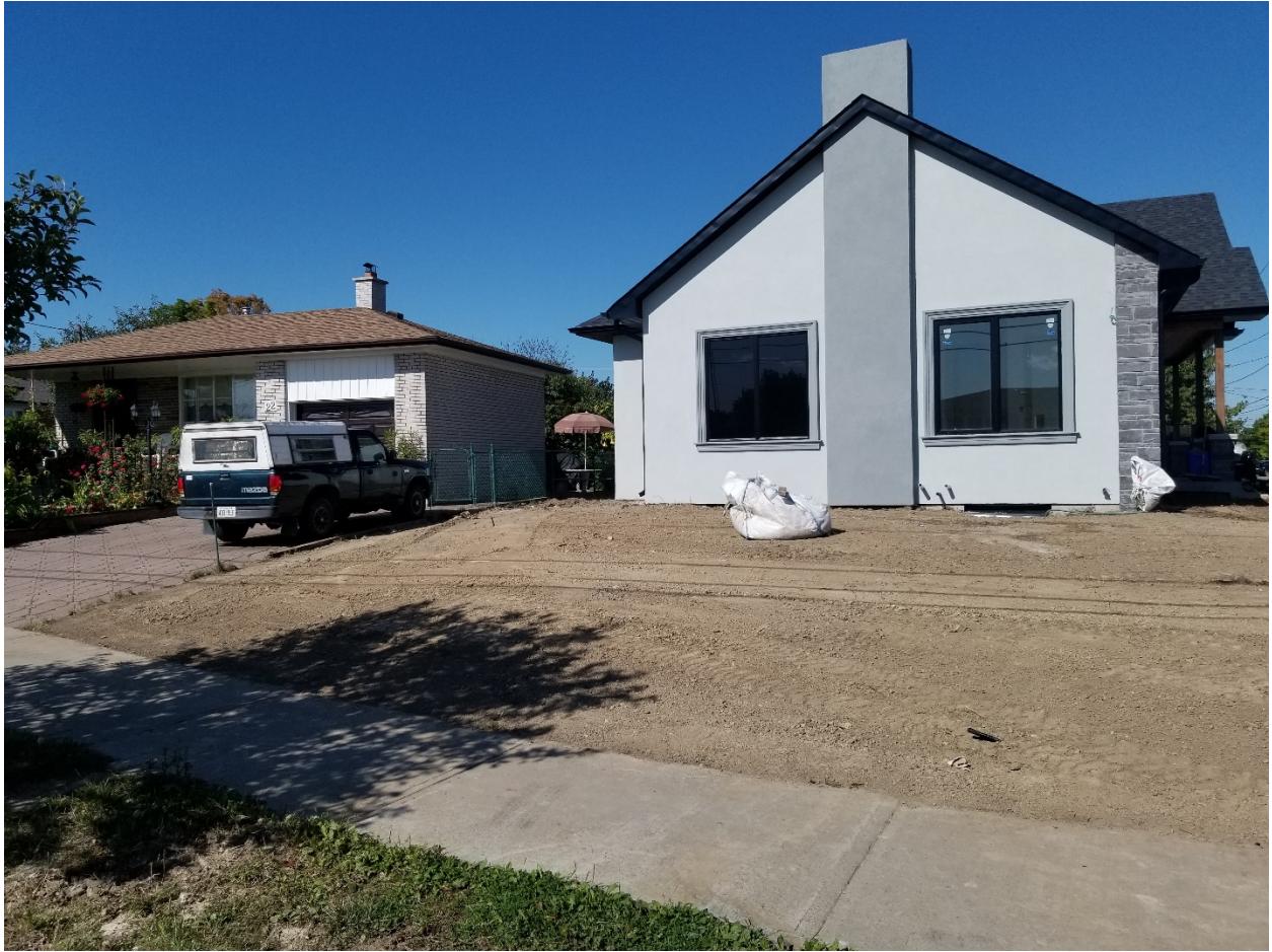
Attachment 4: North West view of 24 Howbert Drive – Rear Yard
