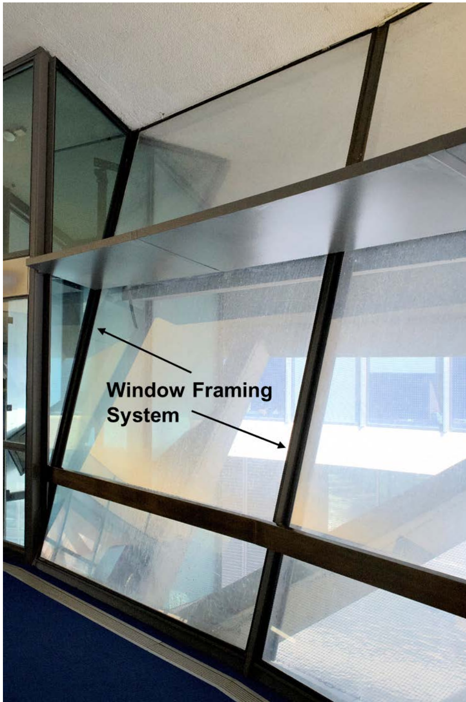
Figure 3: Interior view of existing council chamber window assembly
