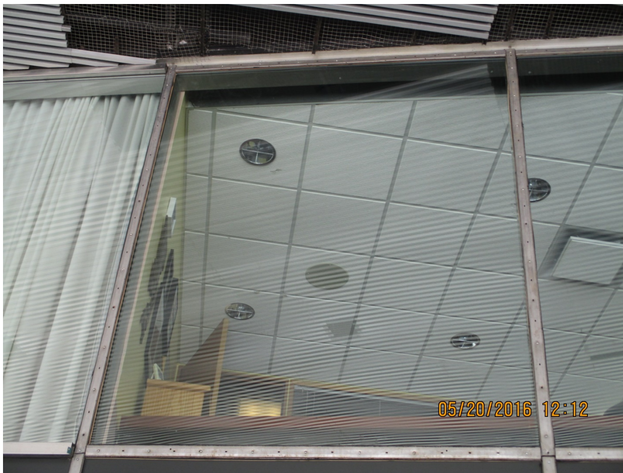
Figure 2: Close-up view of window mock-up
