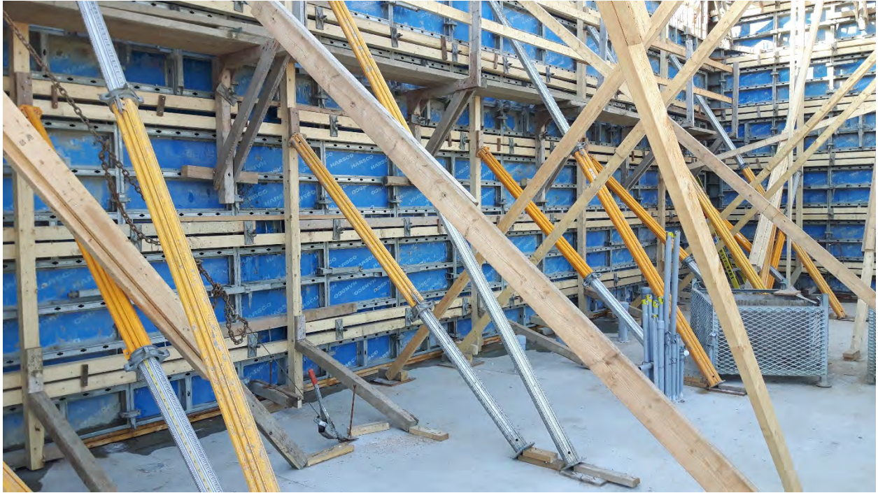
Figure 1 - Concrete Formwork without Cole Engineering Clearance to Proceed
