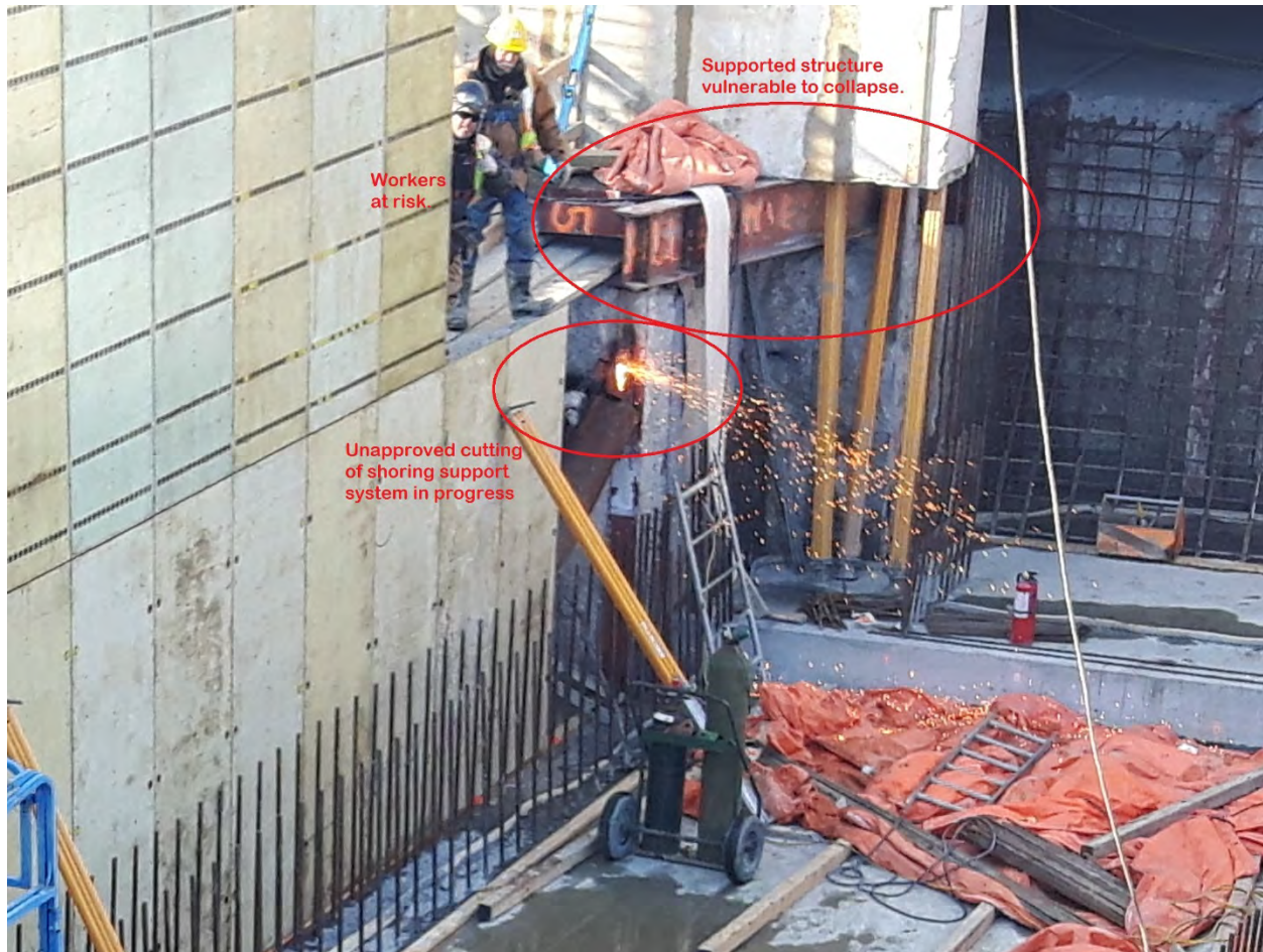
Figure 3 - Shoring System Modification Without Cole Engineering Approval
