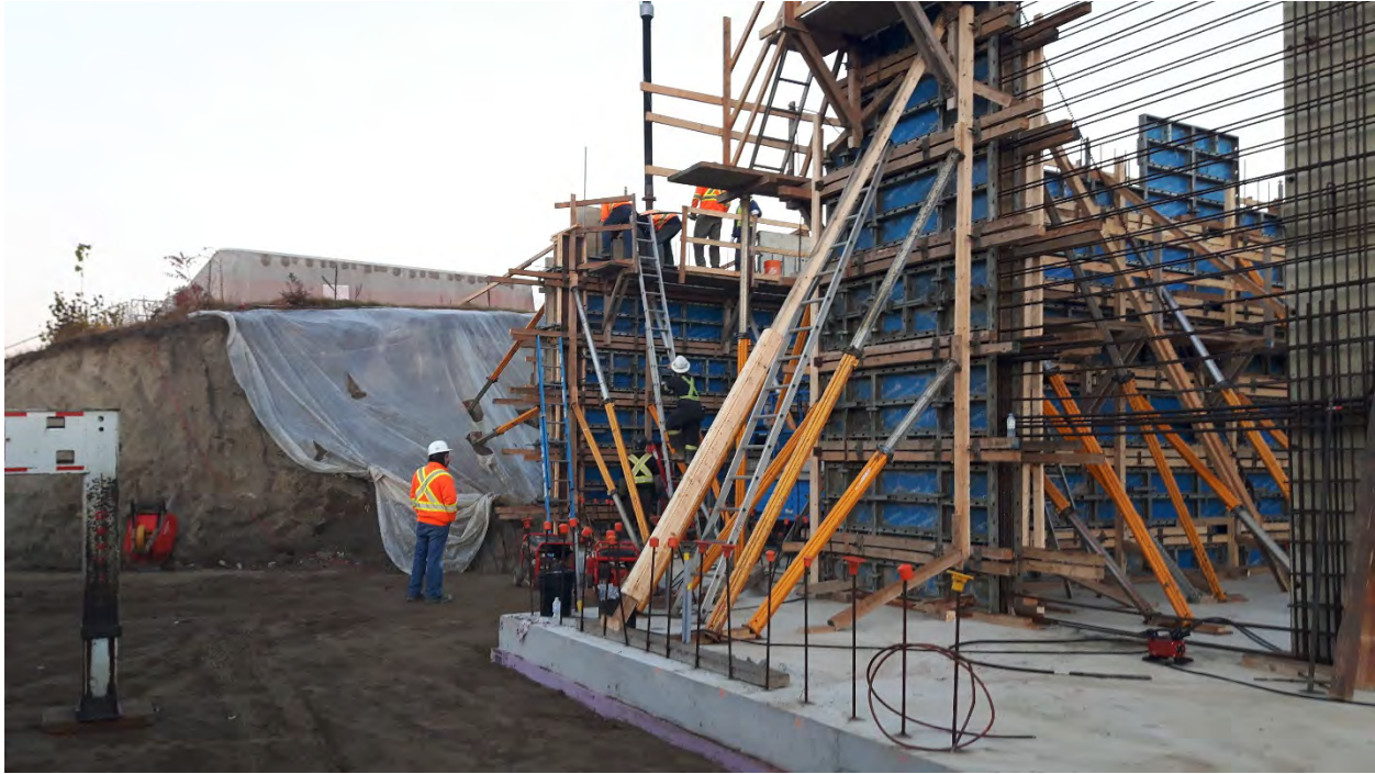
Figure 2 - Formwork and Workers Potentially at Risk
