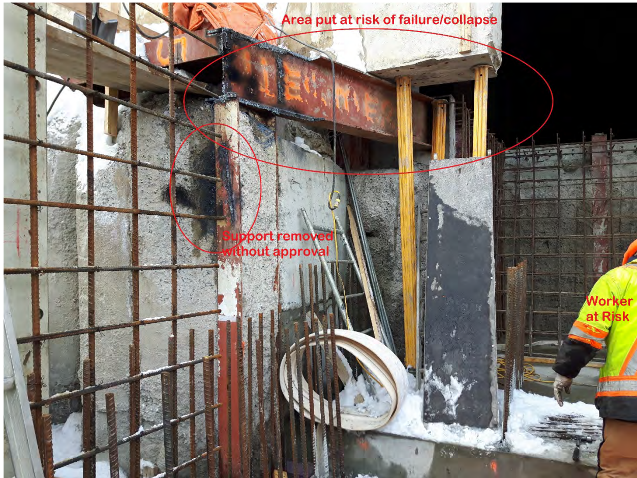
Figure 4 - Modification of Shoring and Workers Potentially at Risk
