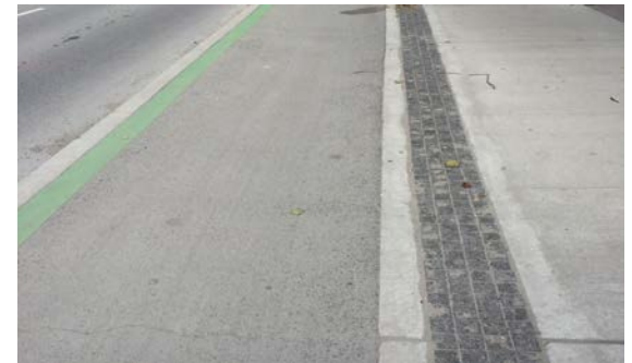
Cane detectable unit pavers between sidewalk and sidewalk-level cycle track
