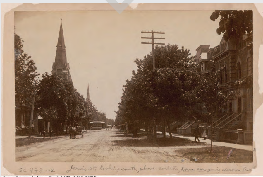
Figure 6: A horse-drawn carriage moves along tree-lined Jarvis street circa 1885 to 1895, which has no visible curb and appears to be surfaced with either gravel or water-bound macadam (crushed limestone). In the background, a horse-drawn bus travels west along Carlton Street. (Source: City of Toronto Archives) 44
