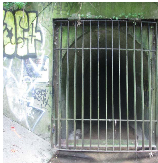
Figure 4: Outfall BC29-3 (formerly L127)
