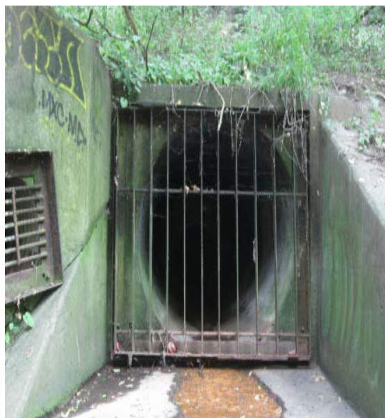
Figure 2: Outfall BC29-1 (formerly L125)
