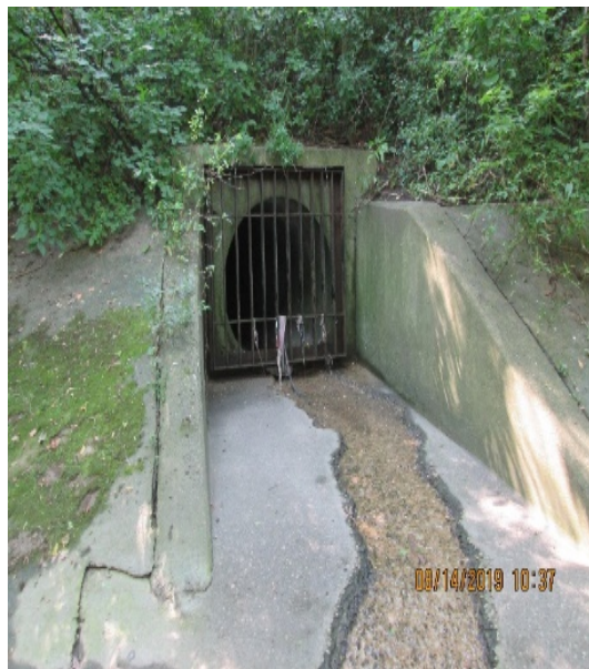
Figure 1: Outfall BC29 (formerly L123)
