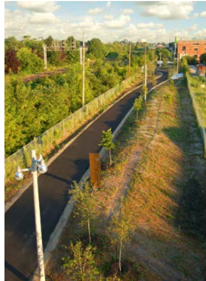
Figure 2. West Toronto Railpath
