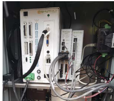
Figure 13: InSync Smart Traffic Signal Control System Installation
