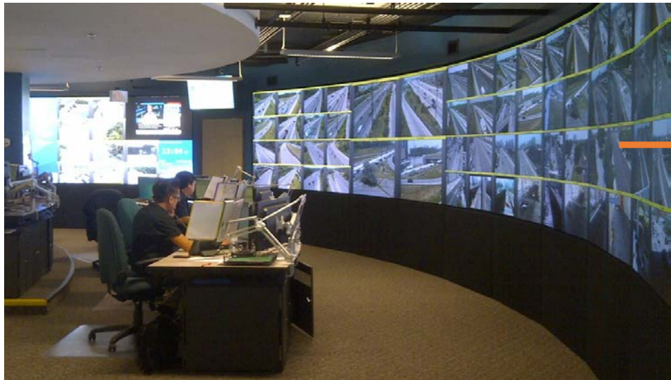
Figure 19: Operators monitoring traffic cameras at the TOC via the Video Wall
